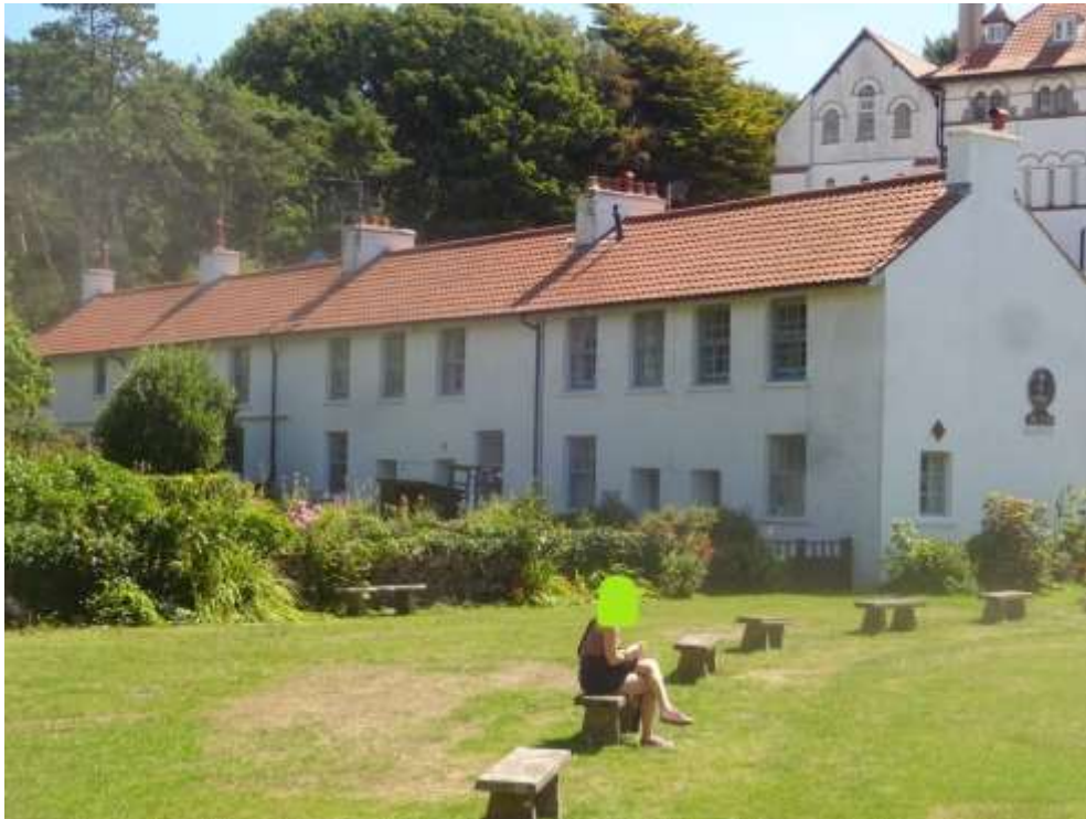
Figure 13 - typical palette of white rendered walls and pan-tiled roofs.
