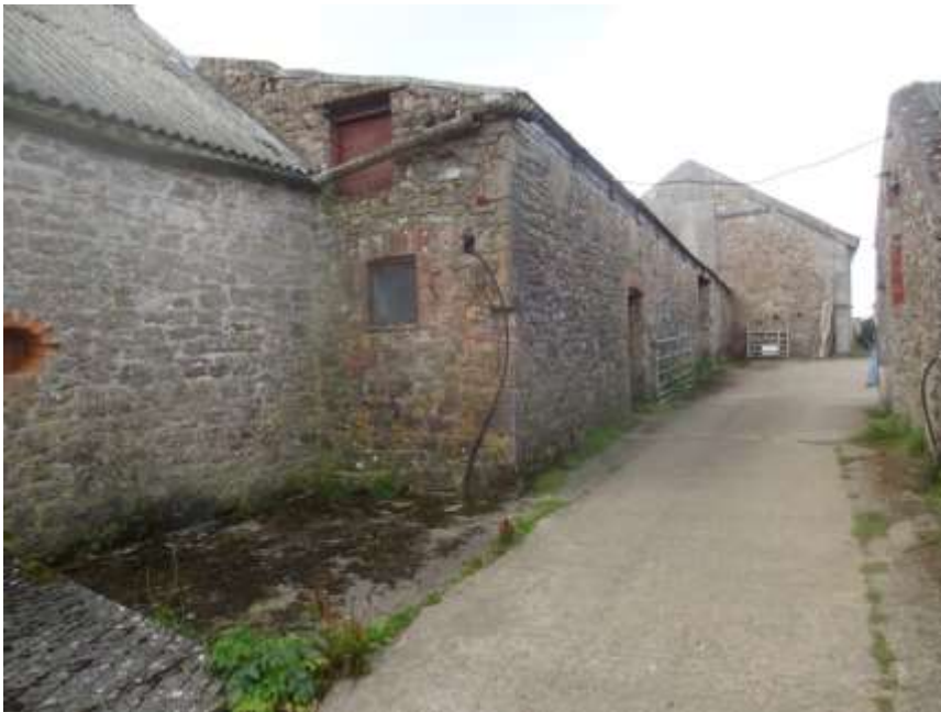
Figure 5 - C19 farm buildings
