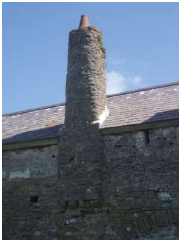
Figure 16 - C16 round chimney, Caldey Priory
