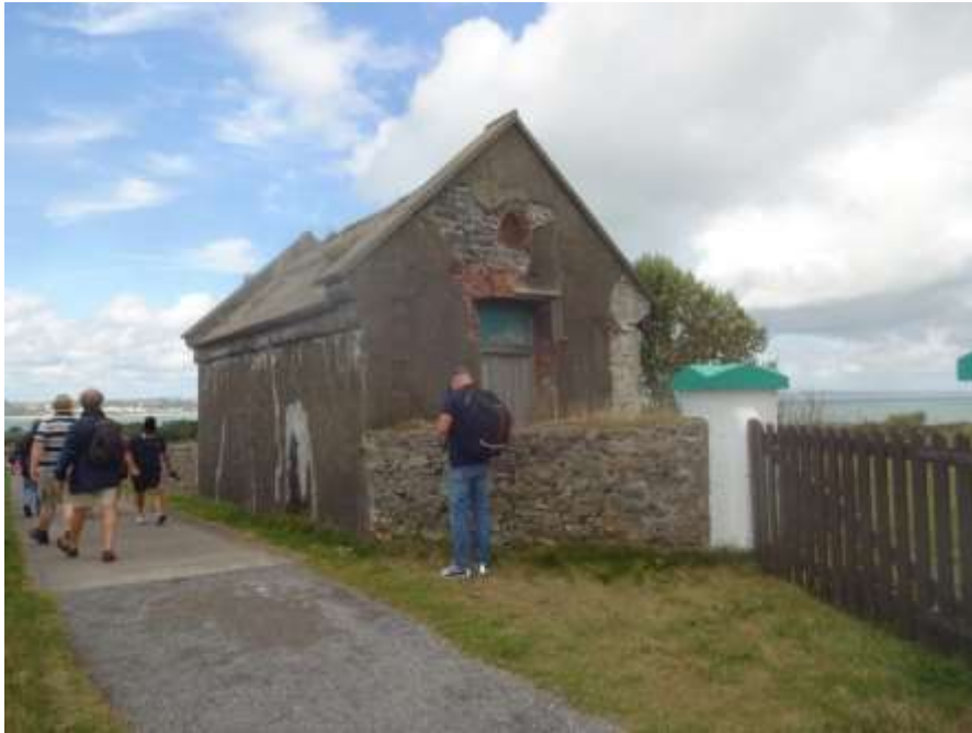
Figure 15 - cement-grouted roof to oil stores
