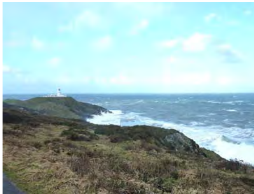
Strumble Head and lighthouse in high winds
