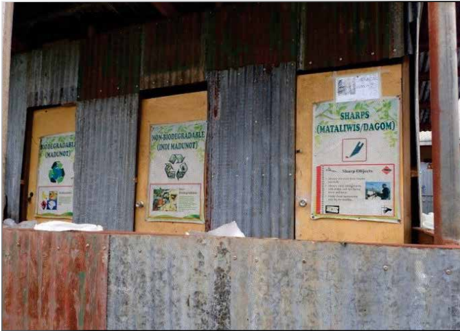
DCGNPH's Materials Recovery Facility.
