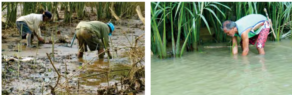
Nipa planting at Barangay Alegria for Sibunag Riverbank Stabilization Project (2015-2016).
