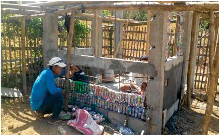
Process of Trash in a Bottle Technology
