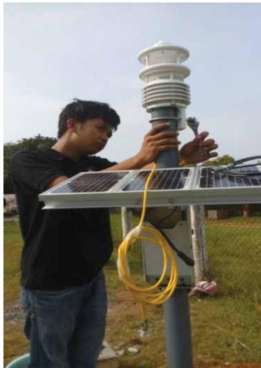
Installation of early warning system.
