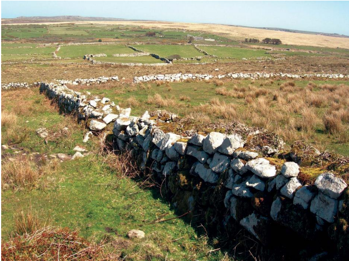
Stone-faced stone walls at Bosporthennis, Zennor.
