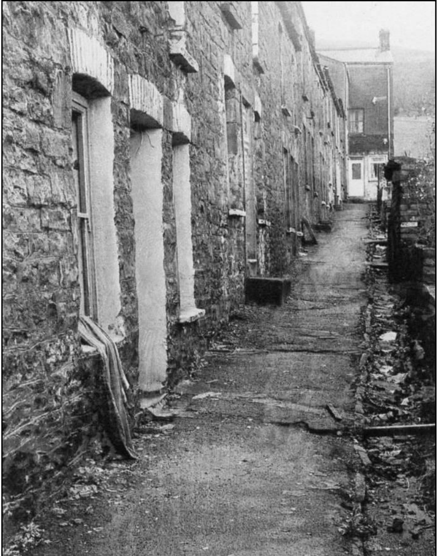
St. David's Square, Abercanaid, built for the local colliers near the No.1 pit. Demolished several years ago.
