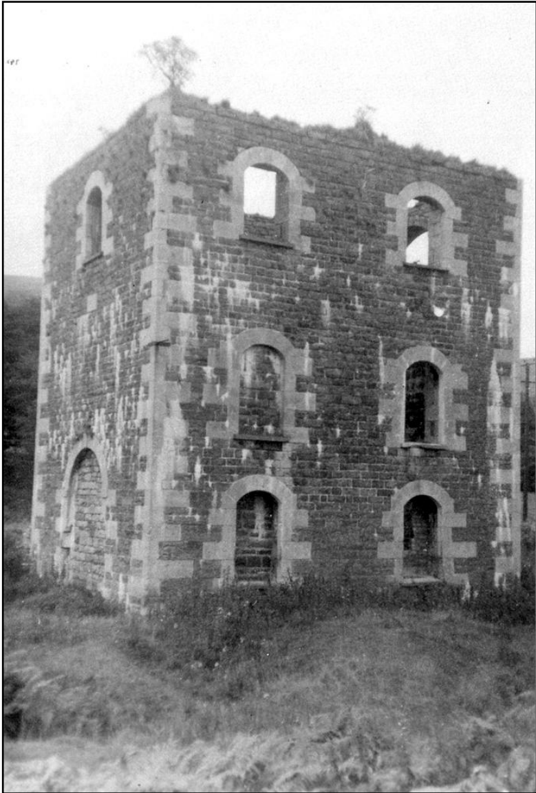
The pumping house at Gethin No.1 pit shortly before demolition. (Photo by Mr. Clive Thomas)
