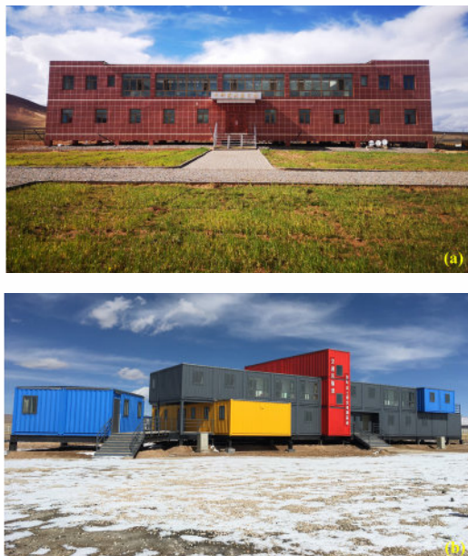
Fig. 16. New qualified national field observational stations for permafrost and permafrost engineering research. (a) Beiluhe Observation and Research Station; (b) Field Observational Station for the Roadway Permafrost Engineering
