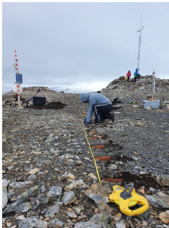
Fig. 45. Setting up the A-ERT monitoring system in Mount Reina Sofia (Livingston Island).
