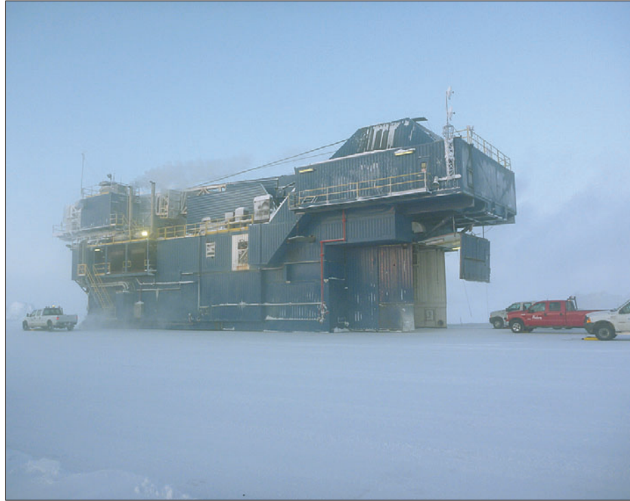
Substructure of Nabors Rig 9ES stopped Feb. 1, 2012, on 2M Pad on its way to Repsol's K-1 drill site at 51 degrees below zero (ambient temp). Rig got underway Feb. 2 when weather warmed up to a balmy minus 22 Fahrenheit. Repsol and other explorers were hindered by one of the coldest winters of record for Alaska's North Slope.
