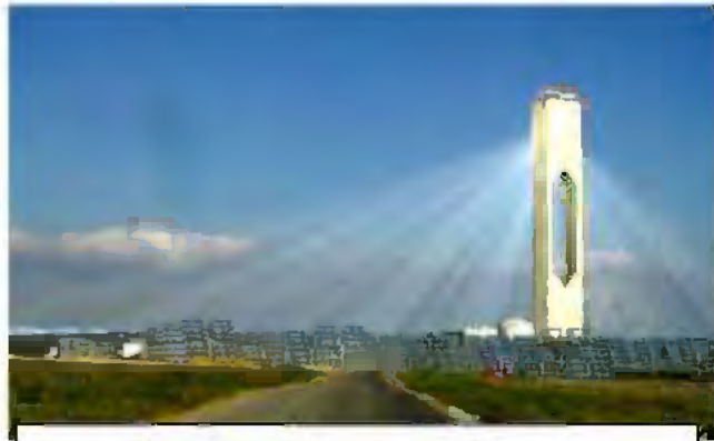
Figure 8: Seville solar power facility ( http://inhabitat.com/sevilles-solar-power-tower )
