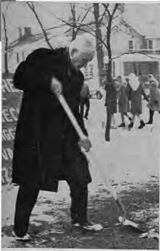
ADMIRAL CLUVERIUS TURNS FIRST SHOVEL
