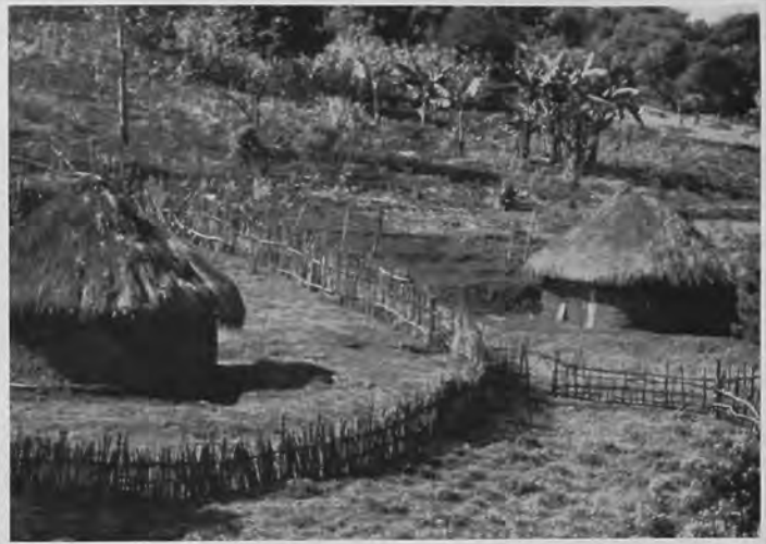
ABOVE: A Kikuyu family homestead with banana trees and a vegetable garden. One house is traditionally occupied by the husband, with houses for each of his wives located nearby. The houses are built of a framework of branches covered with clay. Roofs are grass thatched. Fences keep livestock in at night, safe from thieves and occasional leopards.
