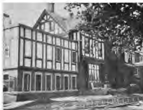
The new addition to the Illinois Delta (Illinois) house is air-conditioned and expands the chapter's resident capacity from 40 to 65.
