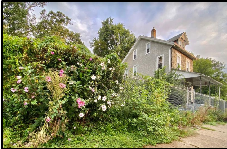
Figure 7. Top: The southeast and northeast elevations. Source: Bradley Maule, 2020. Figure 8. Bottom: The southwest and southeast elevations. Source: Bradley Maule, 2020.
