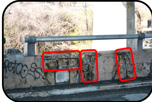
Exposed Rebar
