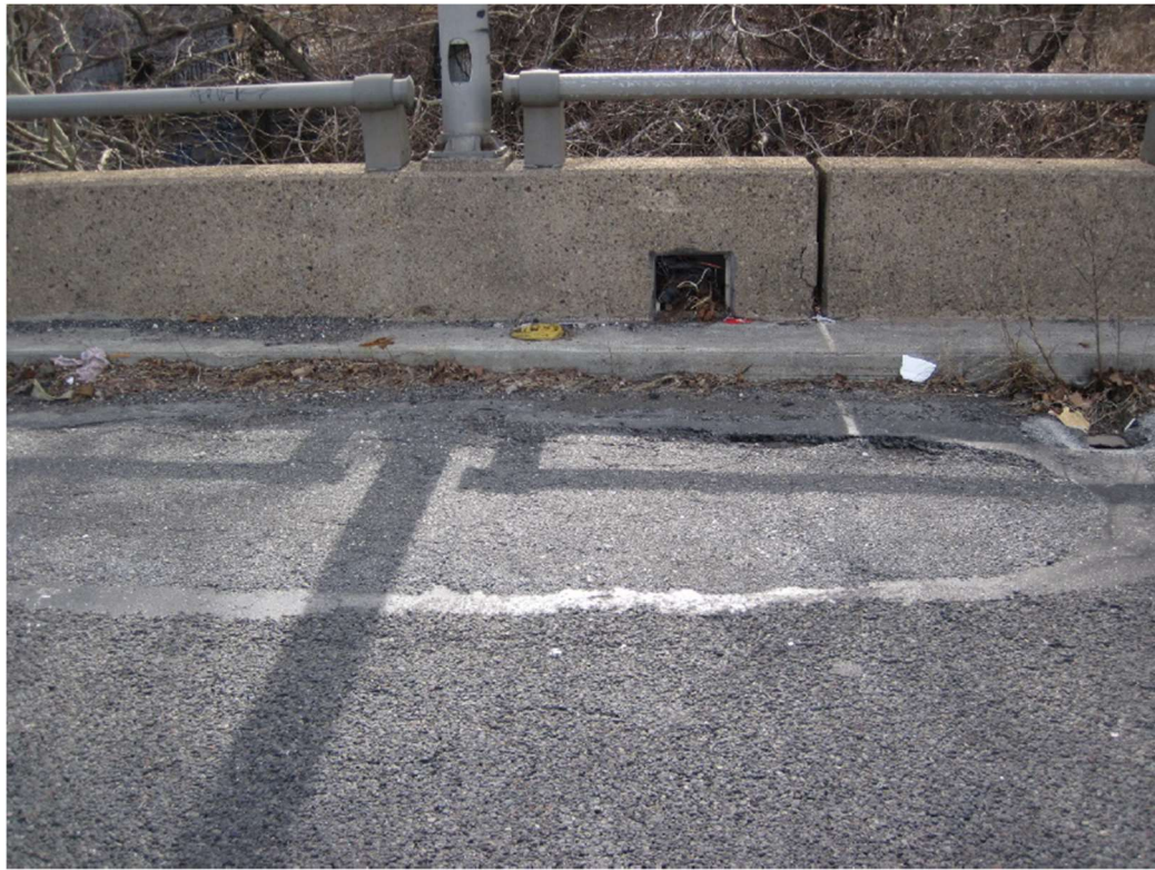
Photo 3 – Existing Safetywalk on Downstream Side and Inside Face of Barrier
