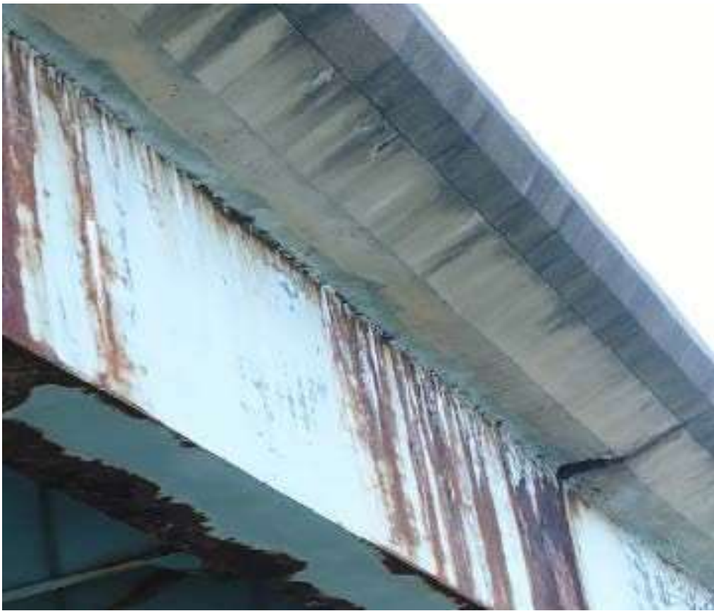
Photo 1 - Existing Girder and Underside of Sidewalk Overhang
