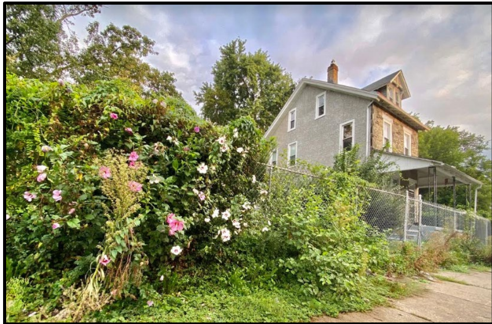
Figure 7. Top: The southeast and northeast elevations. Source: Bradley Maule, 2020. Figure 8. Bottom: The southwest and southeast elevations. Source: Bradley Maule, 2020.
