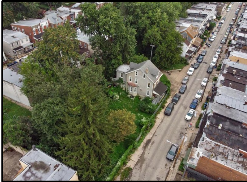
Figure 6. An aerial view of the subject property, showing the southwest elevation in the associated landscape. Source: Bradley Maule, 2020.
