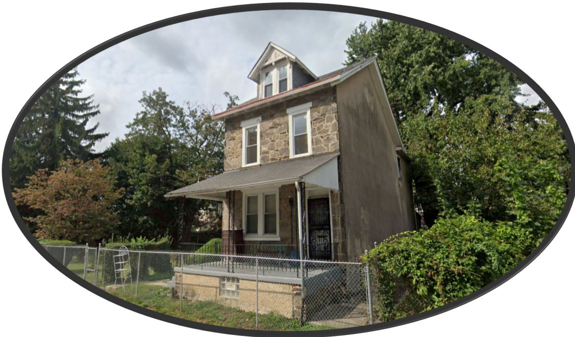
Figure 1. The primary (southeast) elevation of the subject property. Source: Google, 2019.
