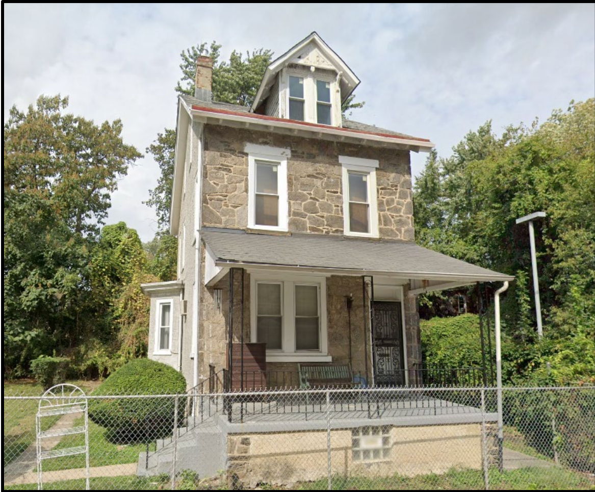
Figure 5. The primary (southeast) elevation. Source: Google, 2019.
