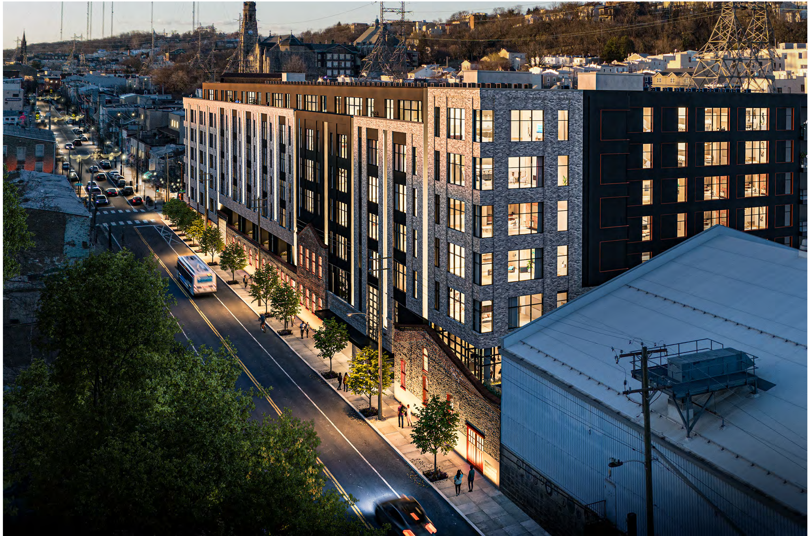
View looking Northwest on Main Street
