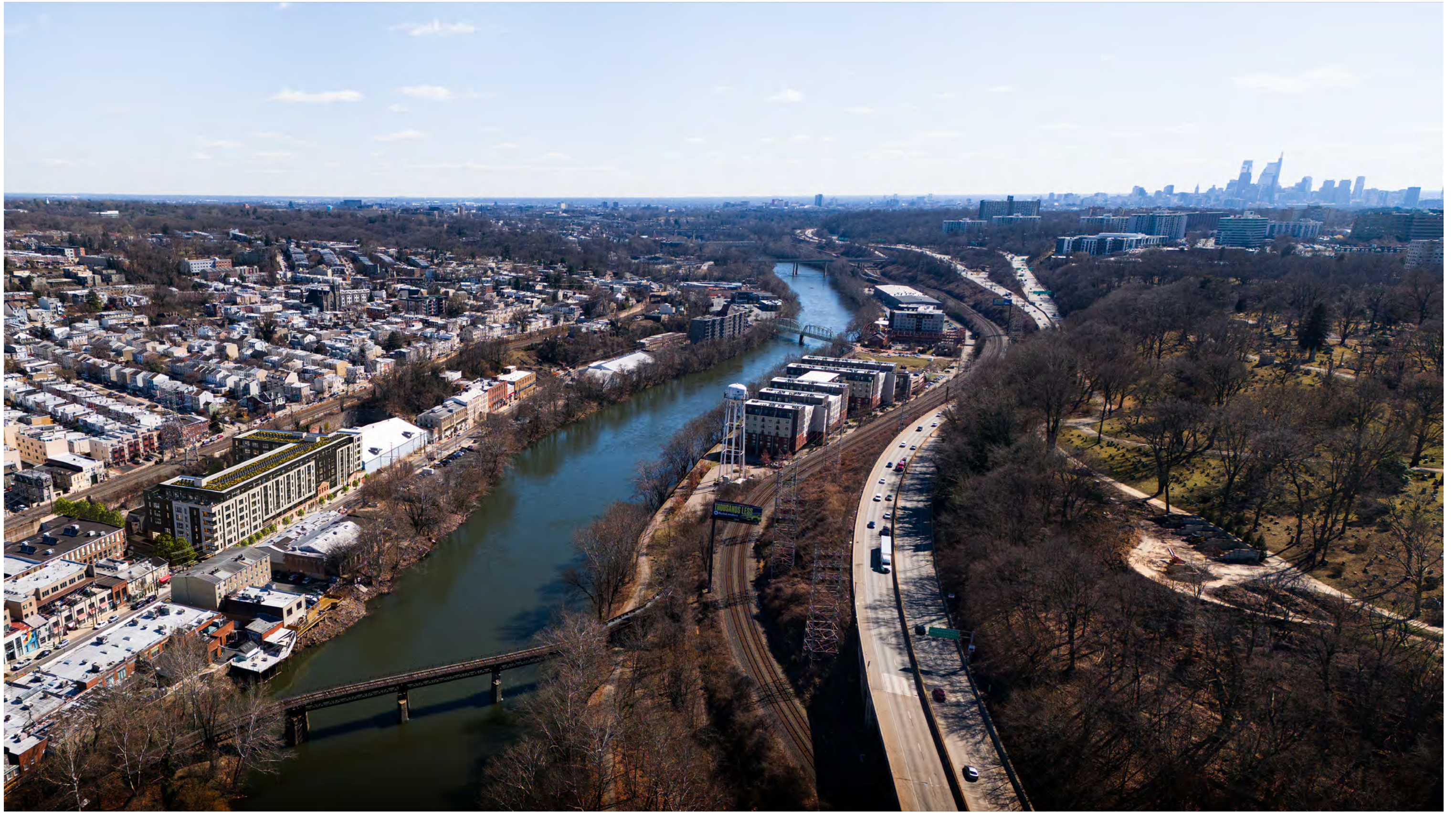
Aerial View looking Southeast
