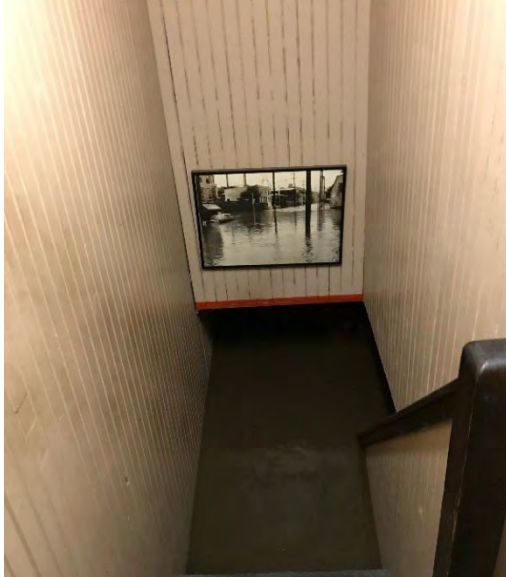
Figure 6: Flood waters entering existing office stairwell.
