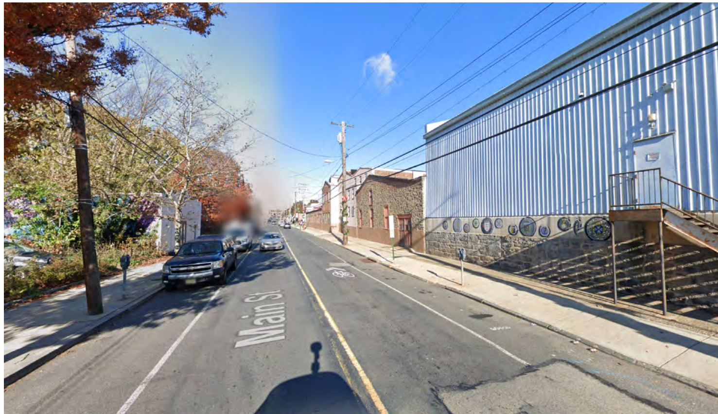
7 View of Site from Main street looking West
