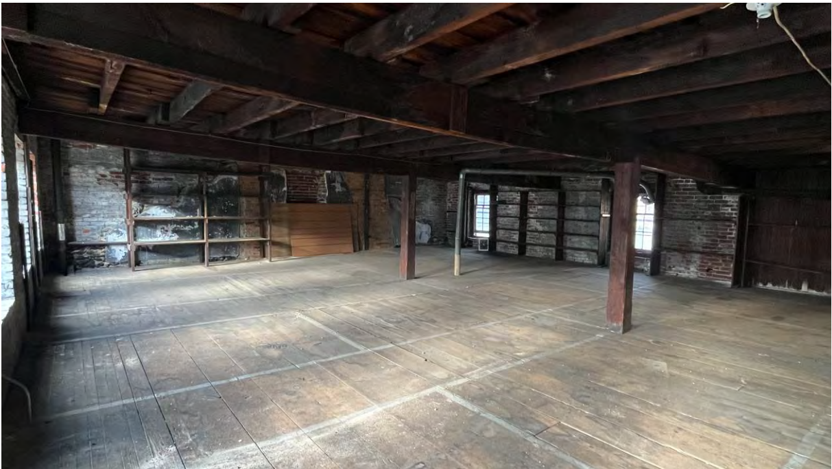
Third floor of office space – low ceilings
