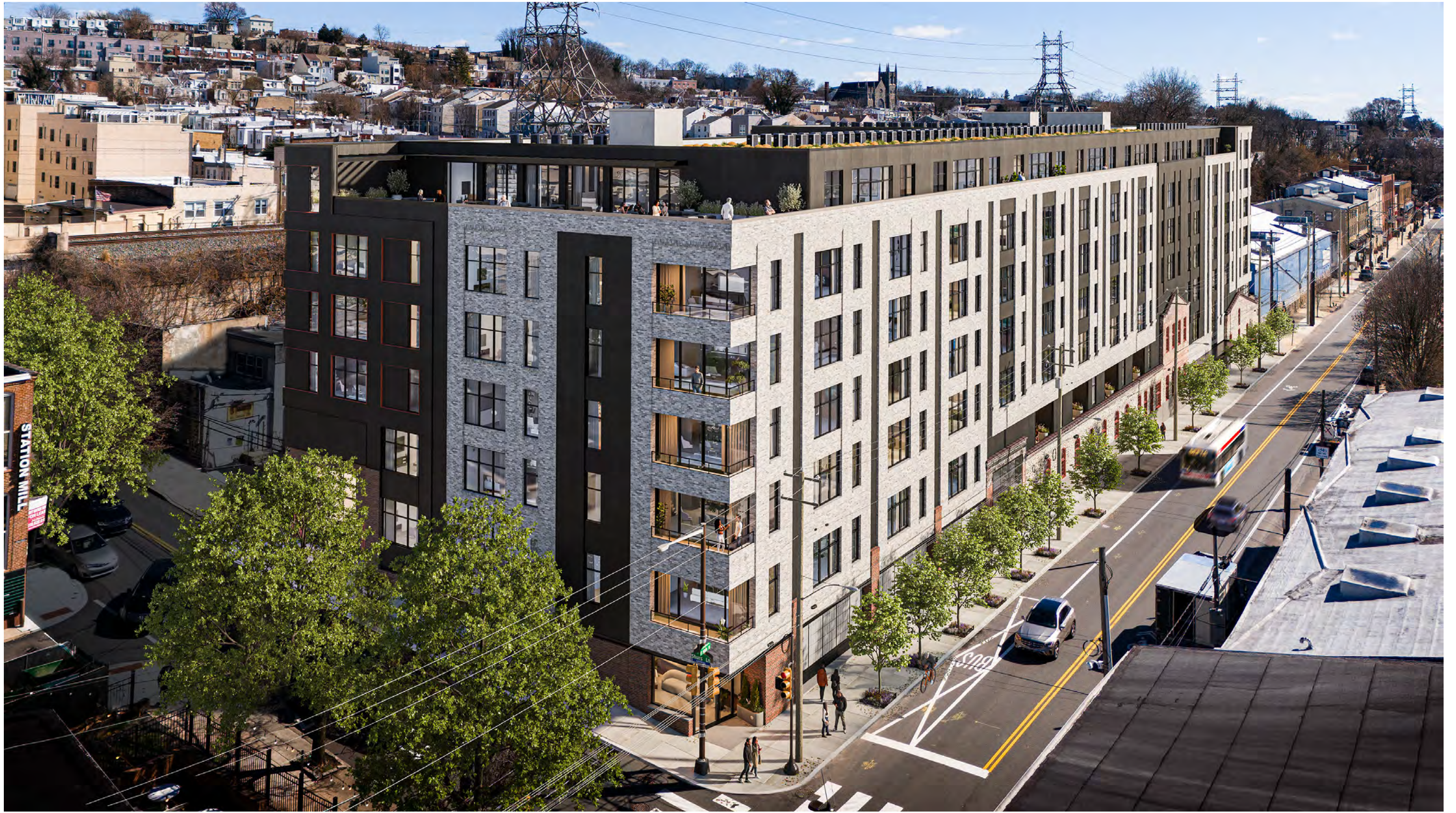
Aerial View looking Southeast
