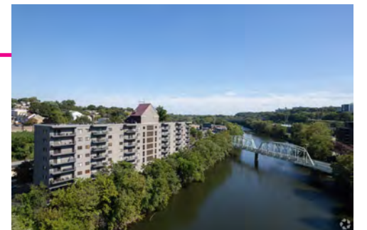
BridgeFive Condominium 3750 Main Street, Philadelphia 7 Stories - 60 Units
