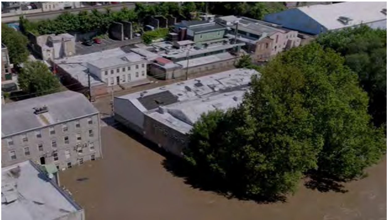
Figure 10. Hurricane Ida flooding in 2021. The photograph shows the water level at the first-floor porch roofline at the office building and mid-way up the large windows in the one-story industrial structure, roughly 10 feet above grade.
