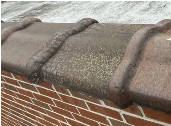
16 Existing Terracota Coping
