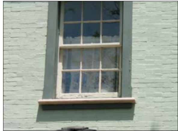
Repair joints to match.
