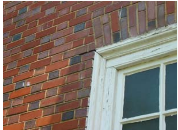
Match mortar repairs to existing color and texture.
