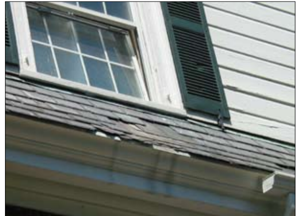
Repair broken or missing slate.
