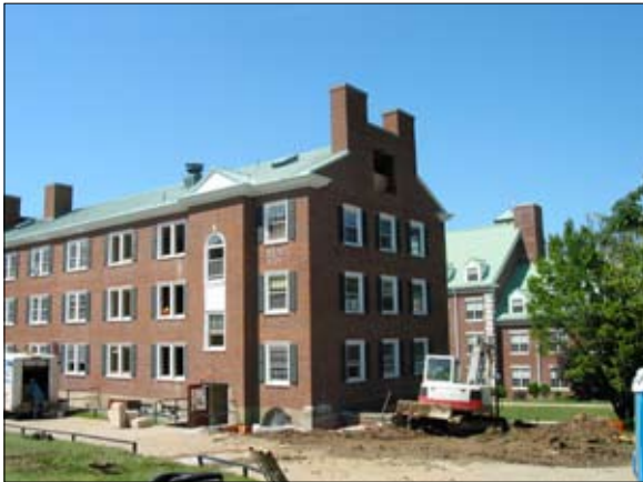
Upper Class under complete renovation.
