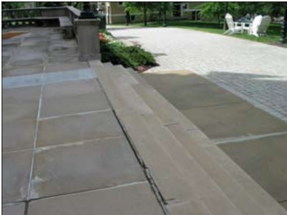
Grout pavers to match stone as needed.
