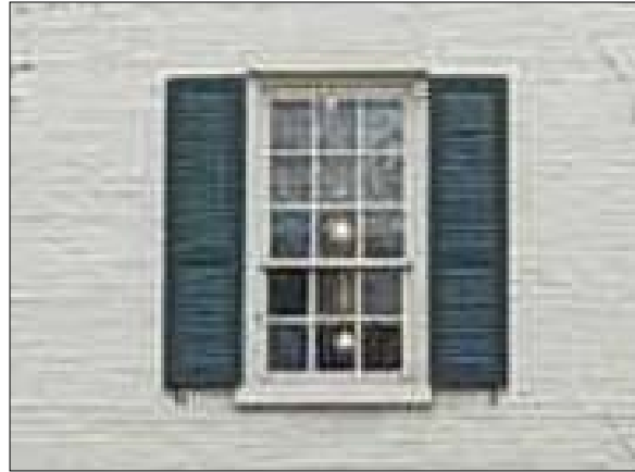
Windows are in fair condition.
