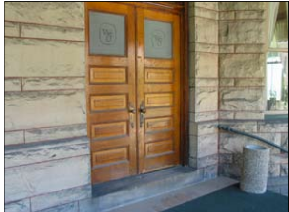
Refinish entry doors.
