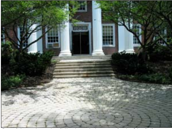
Consider a hand rail that matches period of building.
