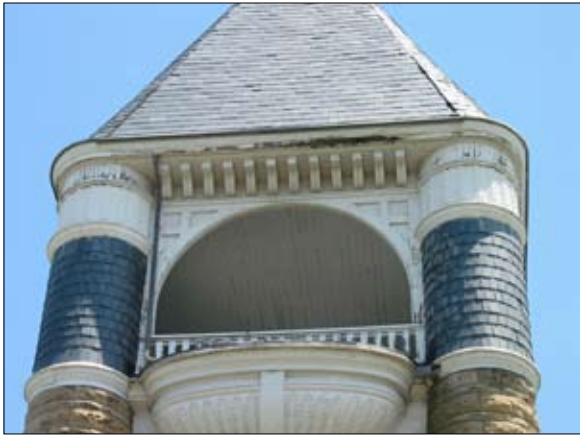
Repair, prime and paint wood detail as needed.
