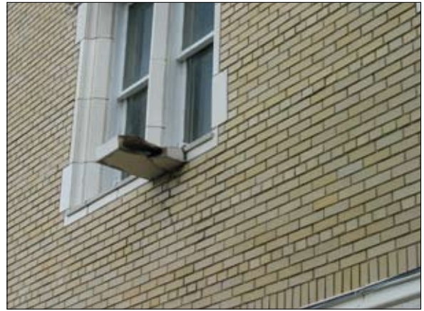
Repair window sills to match original.
