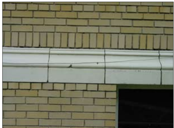
Grout joints in stone copings.
