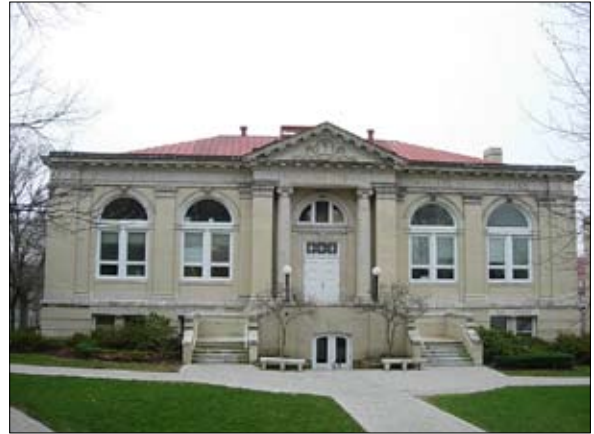
Exterior – Thompson Memorial Hall
