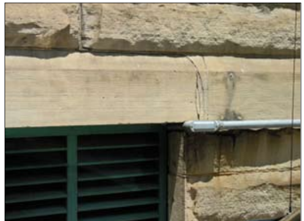
Remove abandoned hardware and repair.
