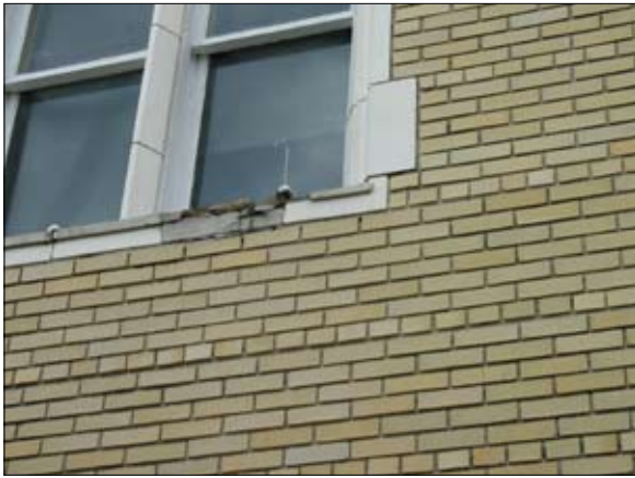
Repair window sills to match original.
