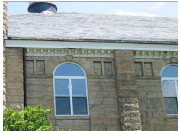
Repair soffit and facia boards as needed.
