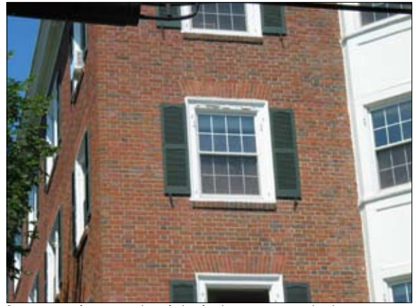
Scrape, prime, and paint windows as needed.
