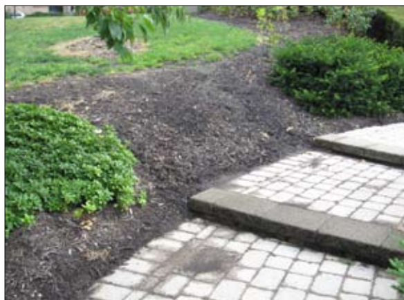
Improper drainage causing mulch to wash out.
