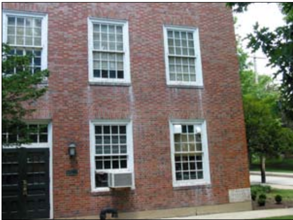
Clean masonry stains caused by old paint.
