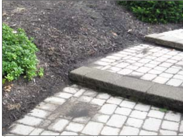
Correct cause of mulch washing out of bed.
