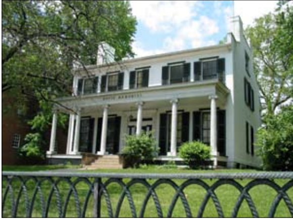
Prune trees back from roof lines
