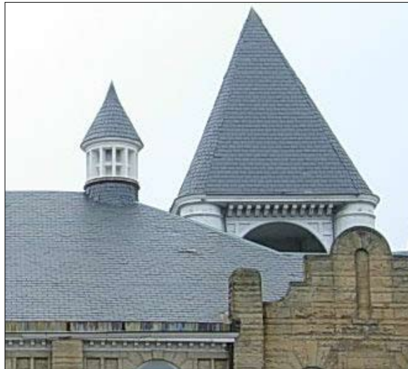
Example of roof coverings – the Wellness Center
