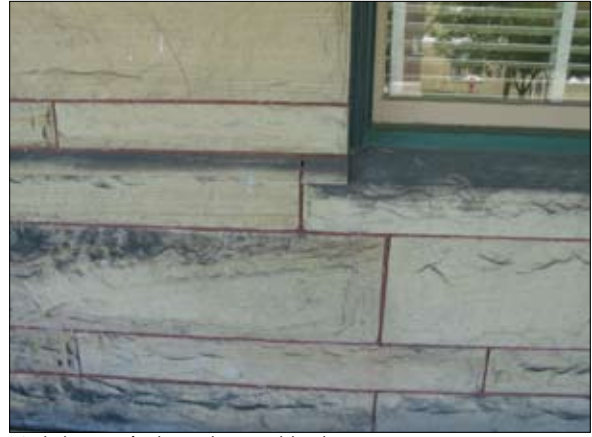
Match repairs to color and texture.
