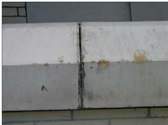
Grout joints in stone capping.
