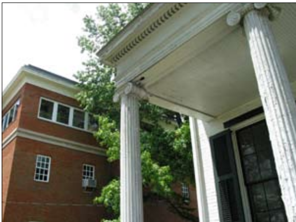
Check flashings and downspouts for obstructions.
