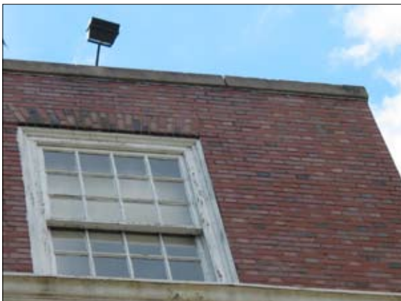
Grout parapet capstones to prevent water damage.
