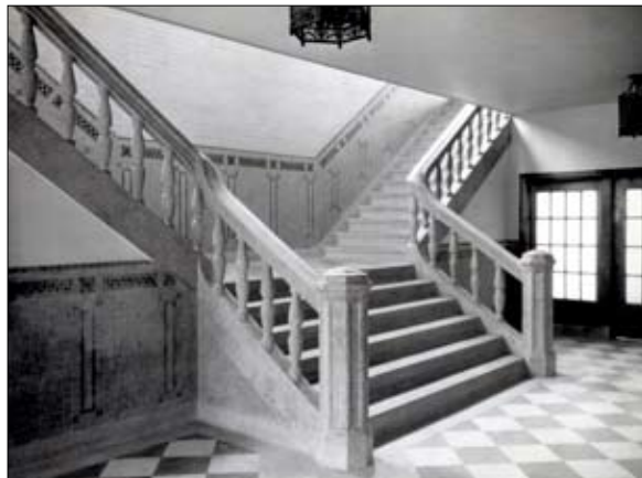
View of original stair, 1927
