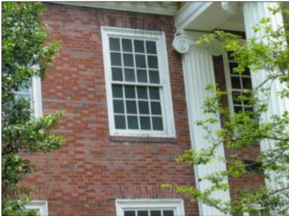
Repair damaged wood, scrape, prime, paint.
