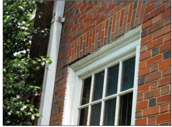
Repair and repaint steel lintels.
