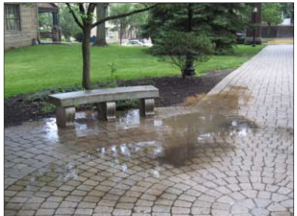
Gutter is spilling onto walkway creating mess.
