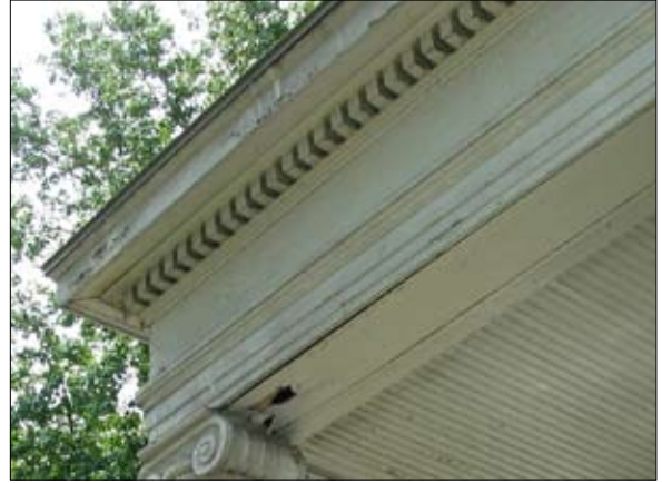
Check flashings and downspouts for obstructions.
