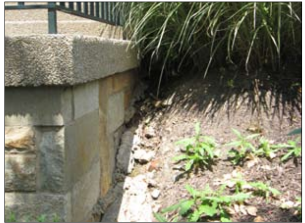
Correct erosion wash along East Beau St.
