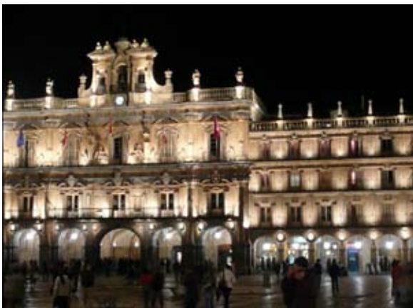
Facade lighting, Salamanca Spain
