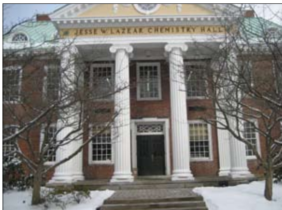
Hawthorns are improperly pruned.
