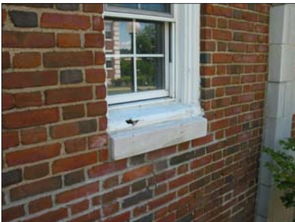
Repair window, scrape, prime, paint.
