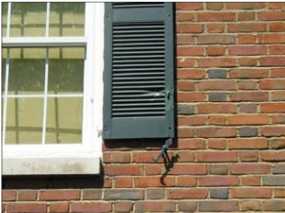
Repair shutters as needed.
