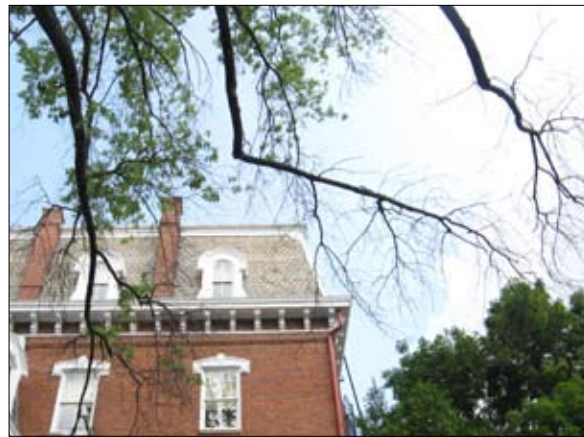
Dead branches are an indication of other problems.
