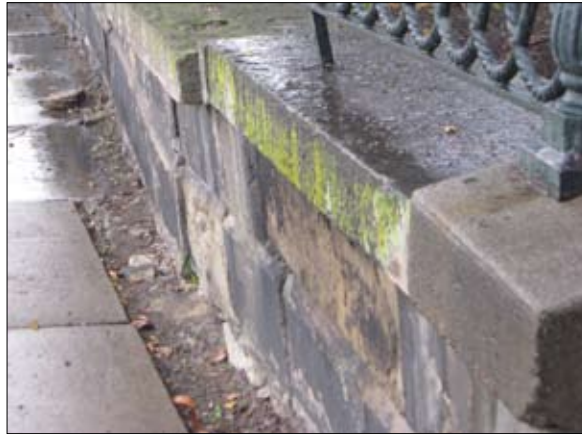
Repair leaning stone wall.
