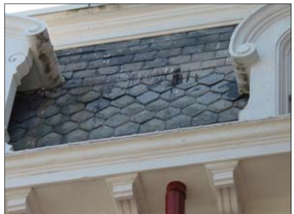
Repair slate, box gutters, downspouts as needed.
