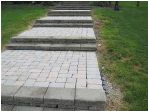
Consider replacing with single-grade walkway.
