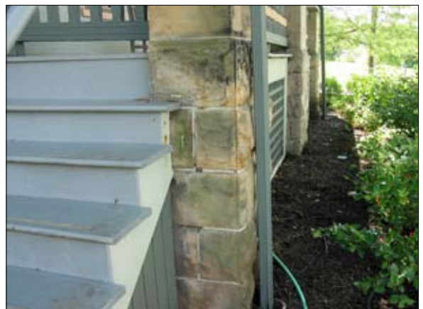
Repair masonry and joints to match original.
