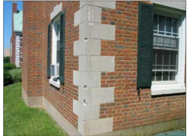
Repair damaged cornerstones.
