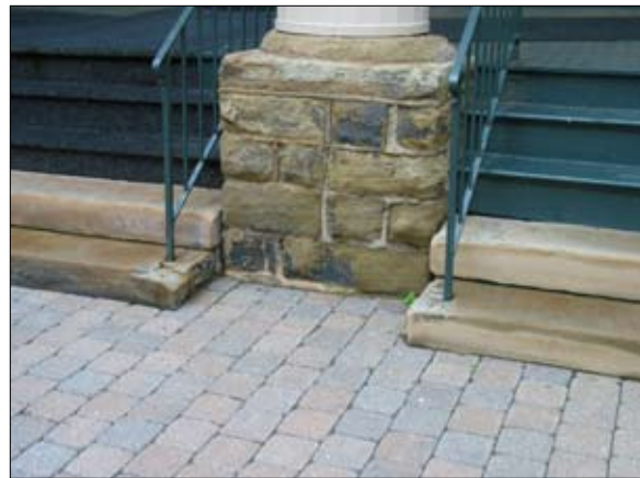
Repairs of mortar should match color and texture.
