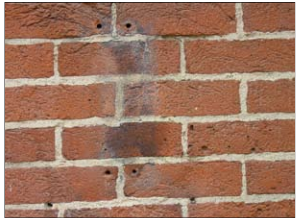
Fill holes in brick to match color and texture.
