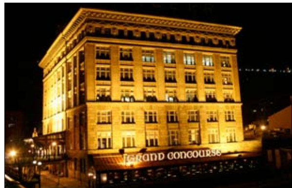
Up-lighting with high pressure sodium lamps lessens the need for more obtrusive street lighting. The Landmarks Building at Station Square, the former Pittsburgh & Lake Erie Railroad main terminal.
