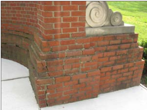
College St. gate damage. Repair.
