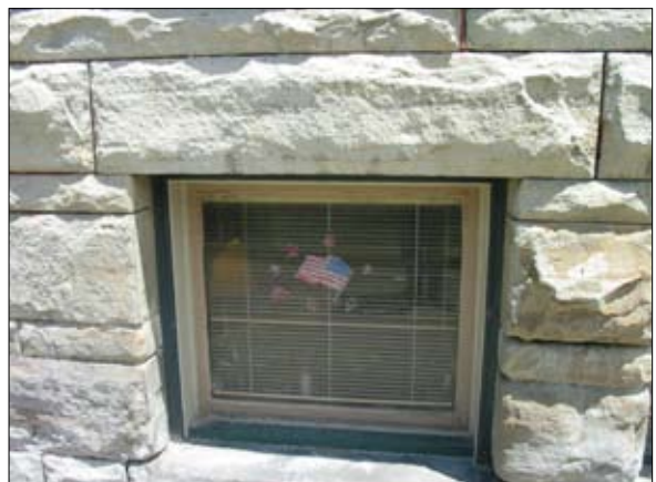
Scrape and prime wood windows as needed.
