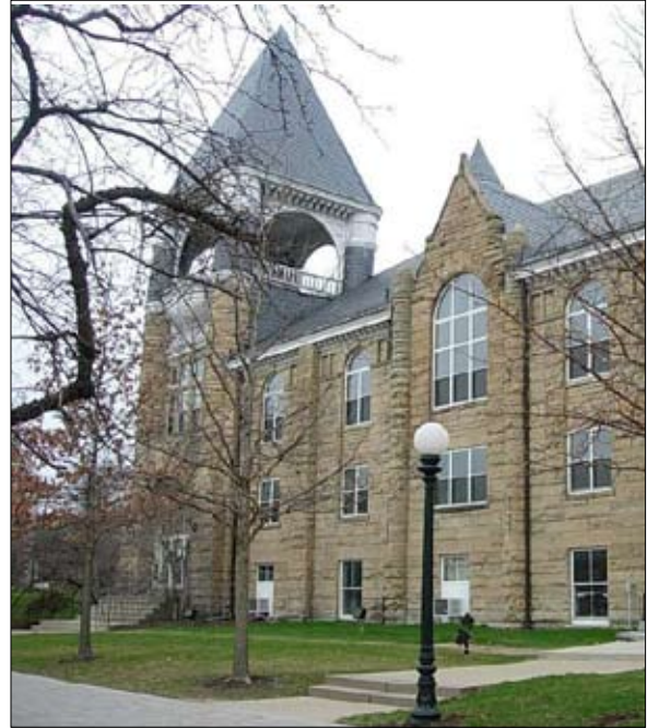
Exterior - Swanson Wellness Center
