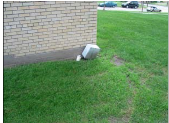
Reconnect junction box to prevent damage.
