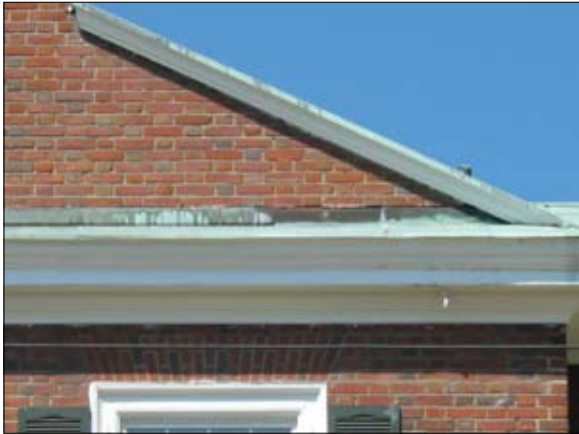
Inspect flashing and slate to prevent water damage.
