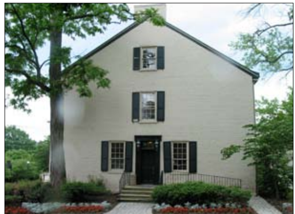
Anchor and level shutters.
