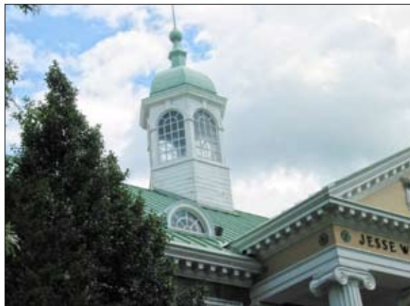
Repair damaged wood, scrape, prime, paint.
