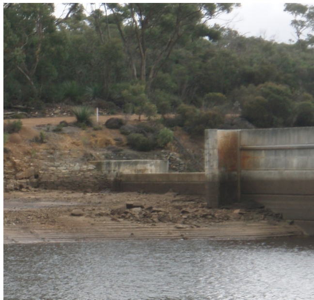
Figure 6. Weir wall at Middle River reservoir viewed from upstream reservoir area. Any restorative works would need to cater for fish passage under lowered reservoir levels such as these that occurred during the G. brevipinnis spawning period in 2010.
