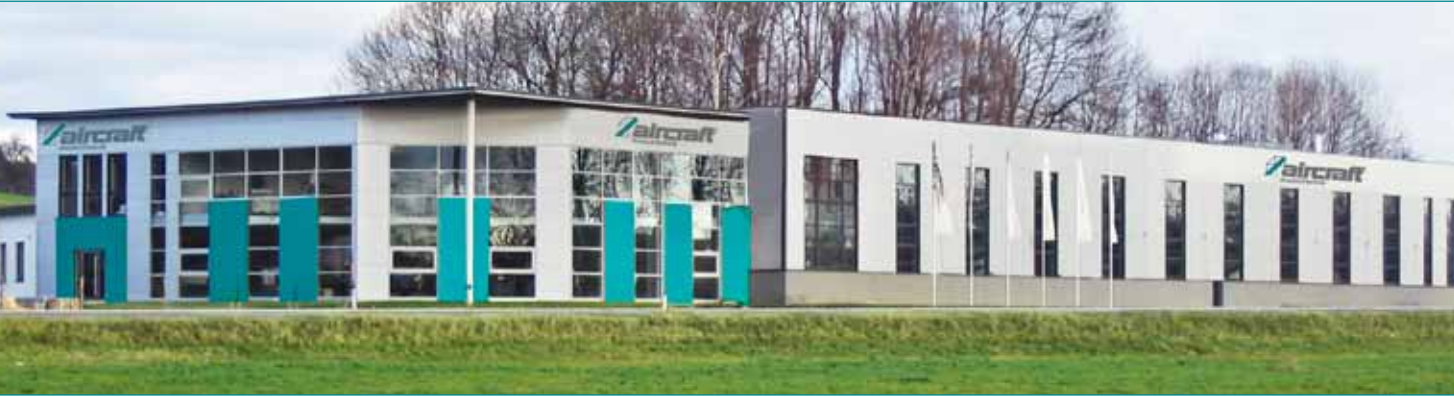
Production and administration building at Hohenzell/Austria
