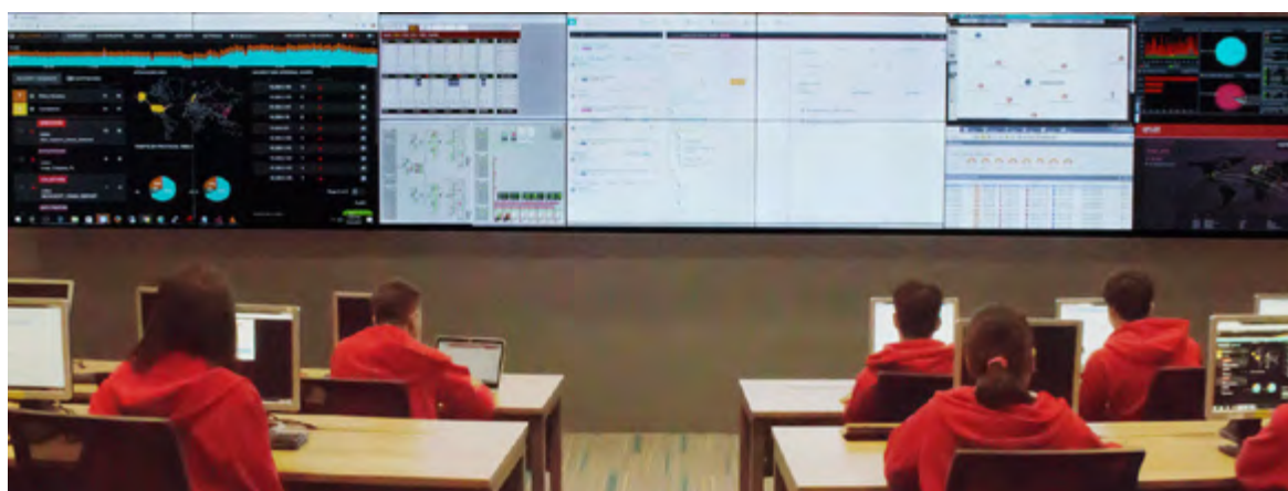
PLDT’s Enterprise Business Group offers a suite of data center, IoT, Cloud, and Cybersecurity services.
