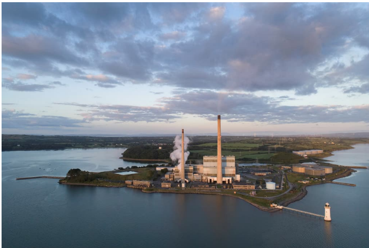
Plate 1.2: Tarbert Power Station. Source: Sean Hartwell Photography, 2020.
