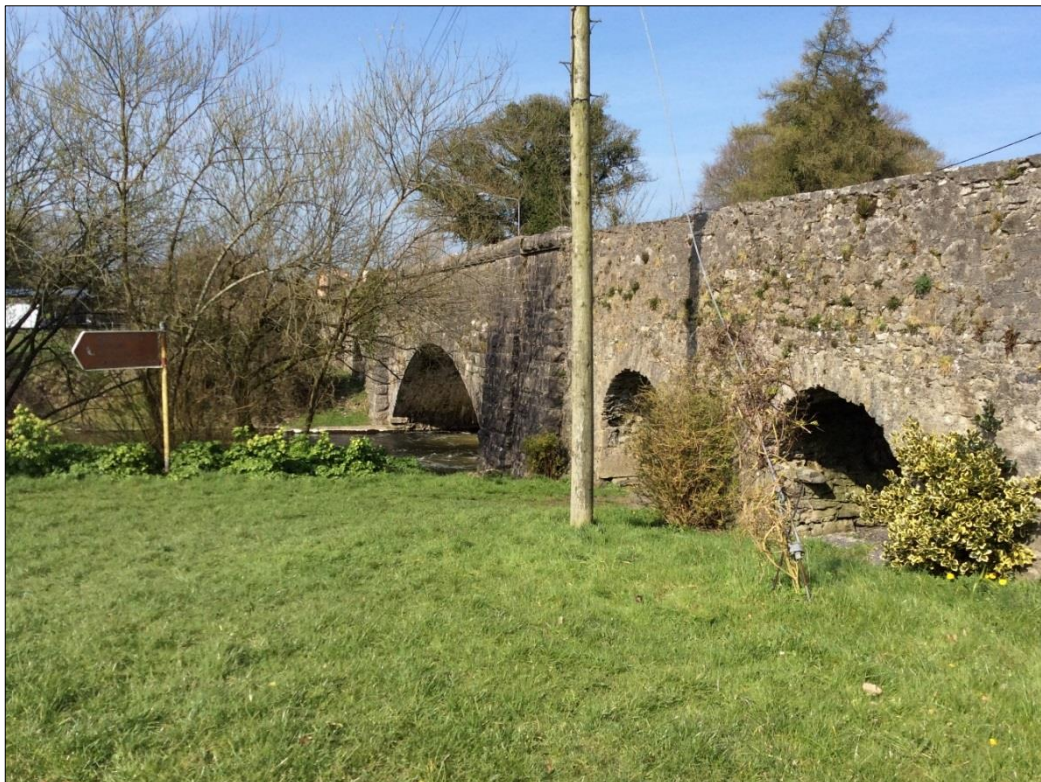
Plate 13-19: Bridge WM001-052/CV041-022 at Finnea, looking NE.
