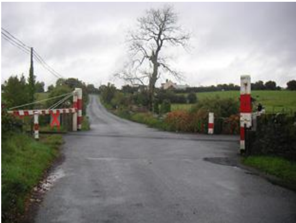
Plate 13-43: Timber level crossing gates (Ref. 019-239) at Farranistick townland along Grid Connection Route (photo from www.buildingsofireland.ie ).
