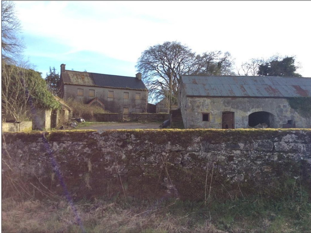
Plate 13-20: View of NIAH structure 15400302 from public road, looking south.
