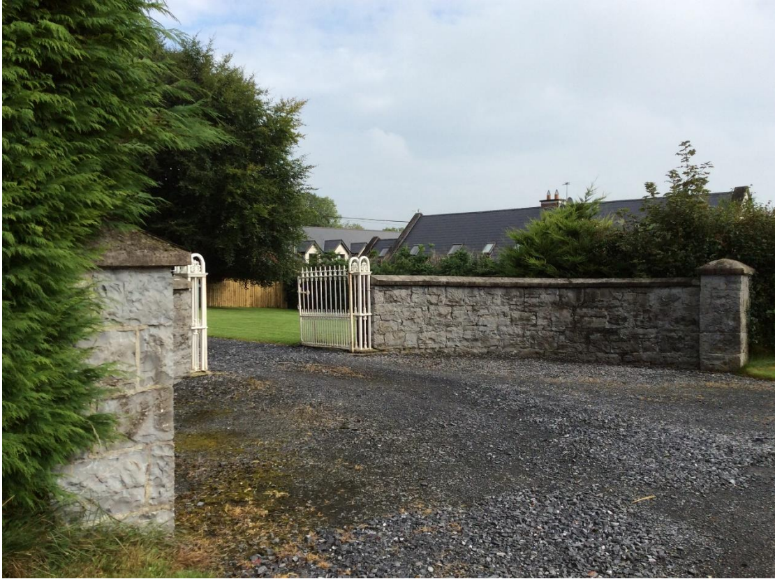
Plate 13-45: Stone wall, piers and cast iron gates at entrance to NIAH 15401915 at Irishtown townland along Grid Connection Route.
