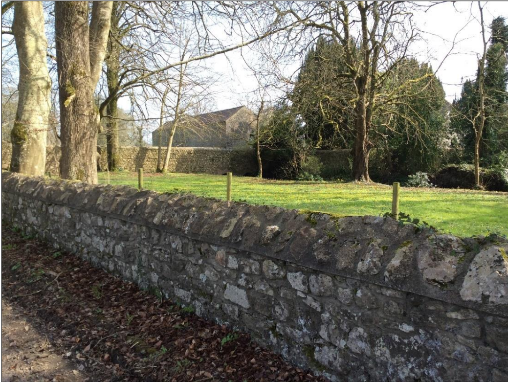
Plate 13-24: Water mills (Reg. 15400305) adjacent to Lickbla House, looking SE from adjacent public road.
