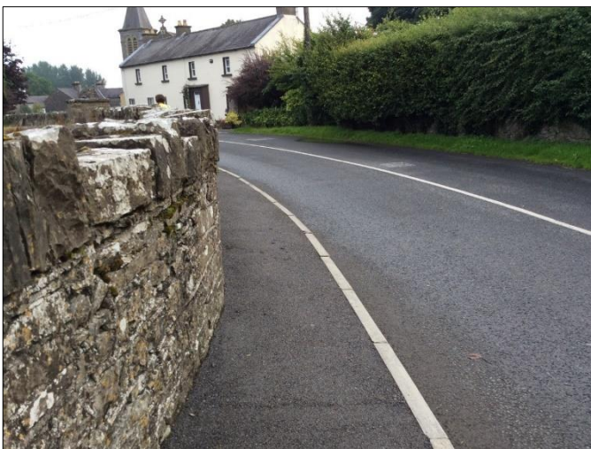
Plate 13-38: Proposed Grid Connection Route where it extends along public road immediately adjacent to graveyard wall, looking north-north-east.
