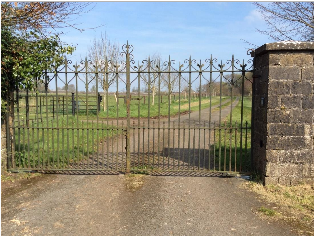
Plate 13-30: Gate and pillars to Turbotstown House adjacent to gate lodge (Reg. 15400332).
