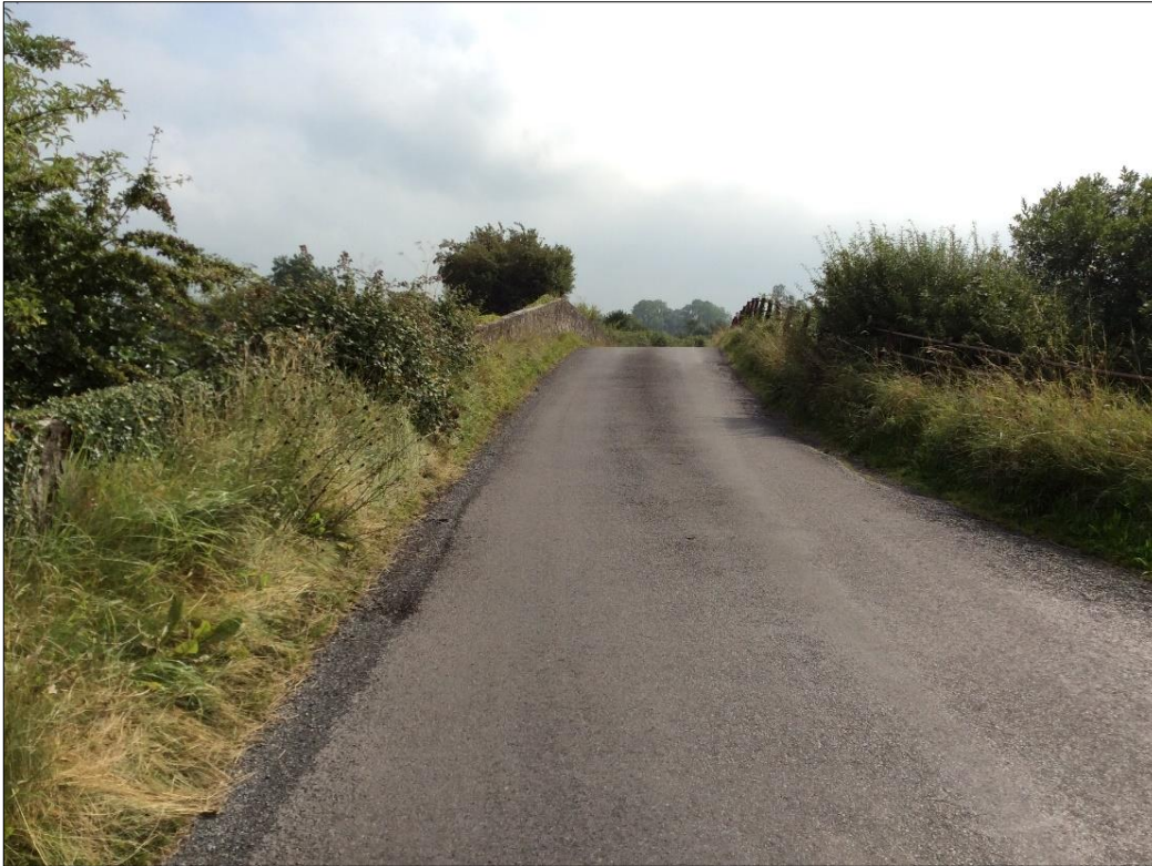
Plate 13-46: Bridge on River Inny along proposed Grid Connection Route at Shrubbywood/Clonva.
