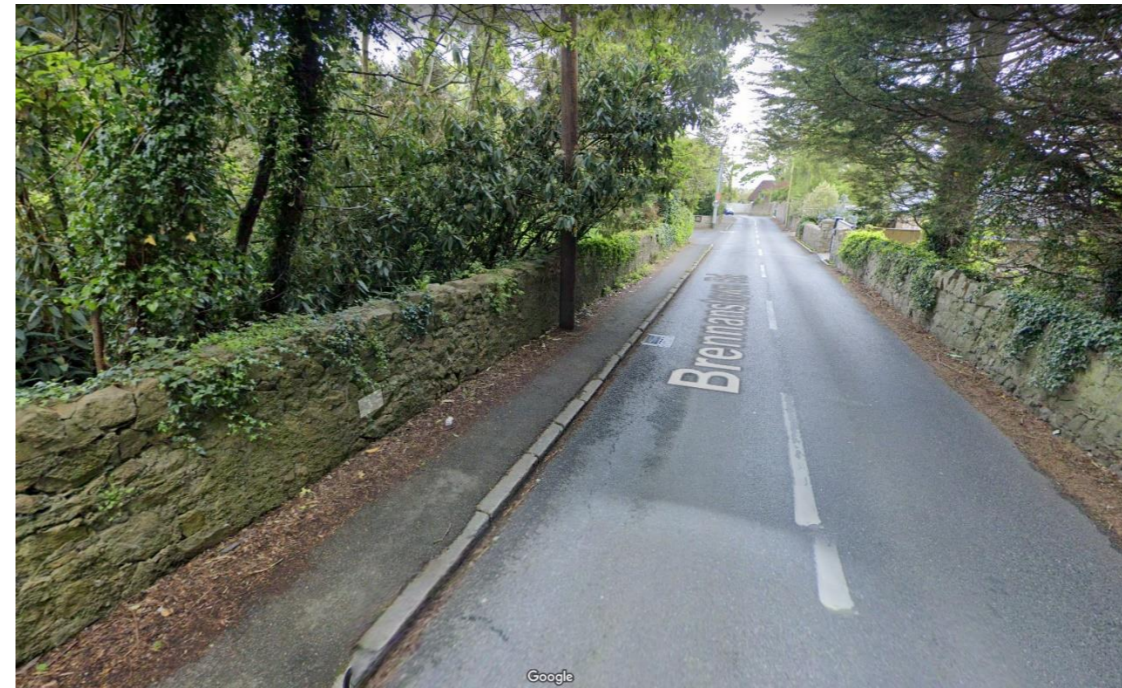
Existing footpath on Brennanstown Road
