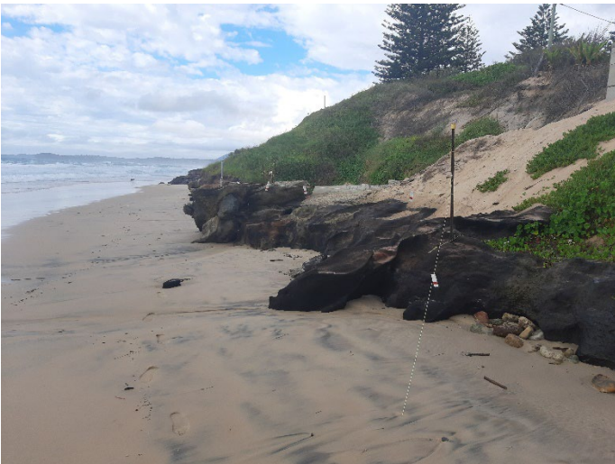
Figure 5: Site of proposed works looking south (5/1/23)
