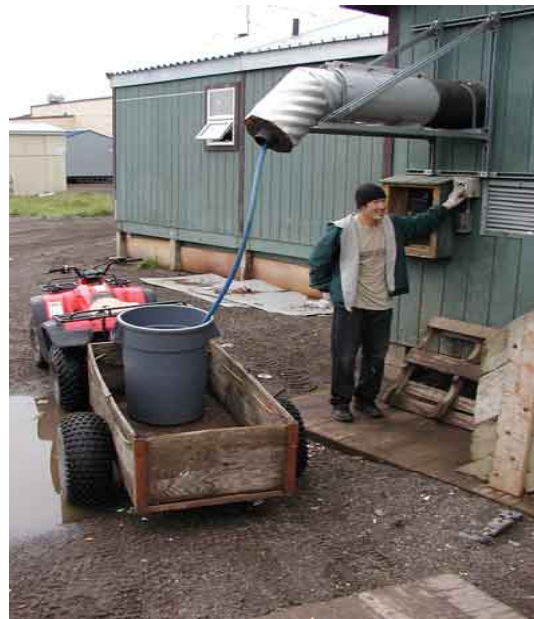
Kivalina washeteria watering point (TNH/URS, 2003)
