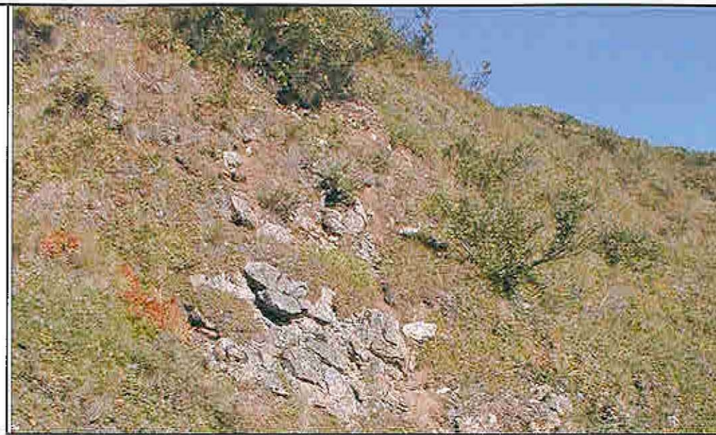
Imnakuk Bluff, Photo 4 Limestone gravel at face at stream channel
