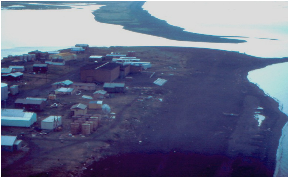
This 1983 photo of Kivalina shows the distance between the village school (the large brown building to the left of center) and the shoreline. The shoreline has now eroded so that the shoreline is a few feet from the school.
