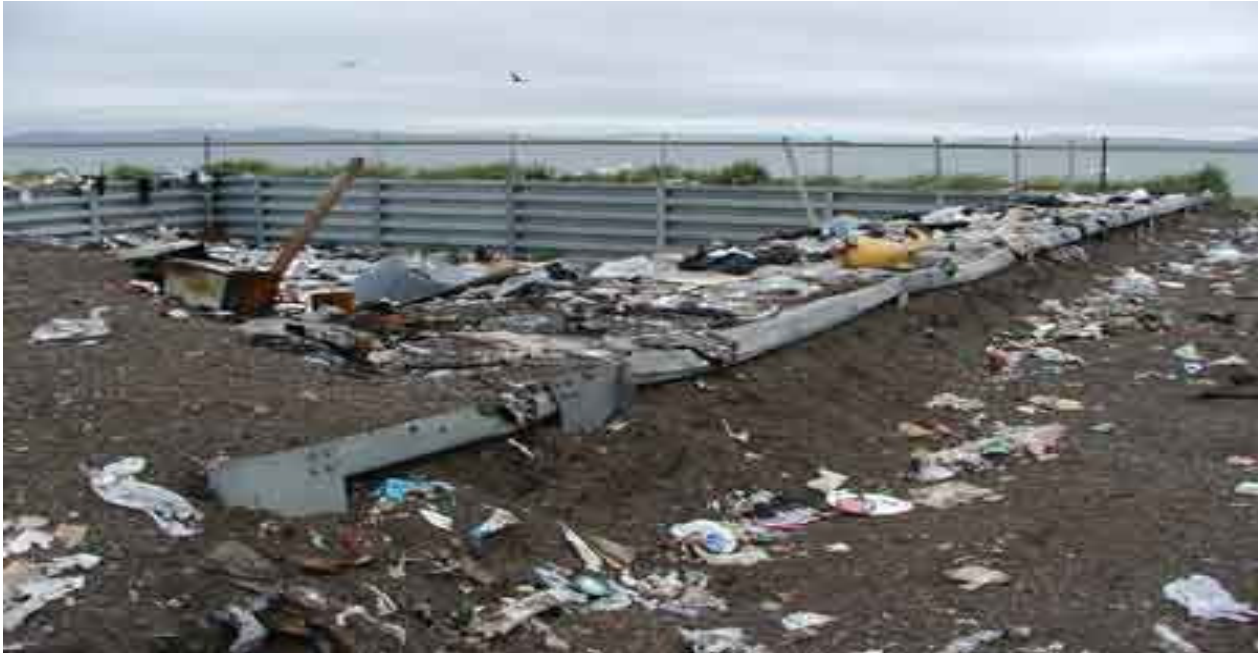
Kivalina honey bucket containment bunker at landfill (TNH/URS, 2003)
