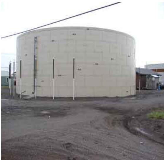
Kivalina water storage tank (TNH/URS, 2003)
