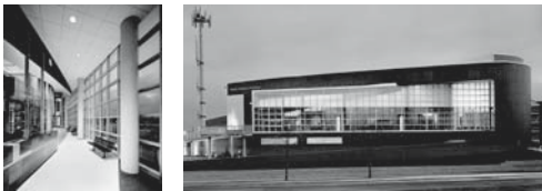
Niles Police Station Niles, Illinois 50,000 square feet
