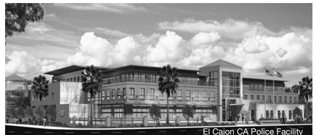
El Cajon CA Police Facility
