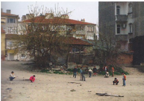
Illegal building surrounded by residential settlement in Istanbul. Photo by Marco Sodano, Cluster, issue 07
