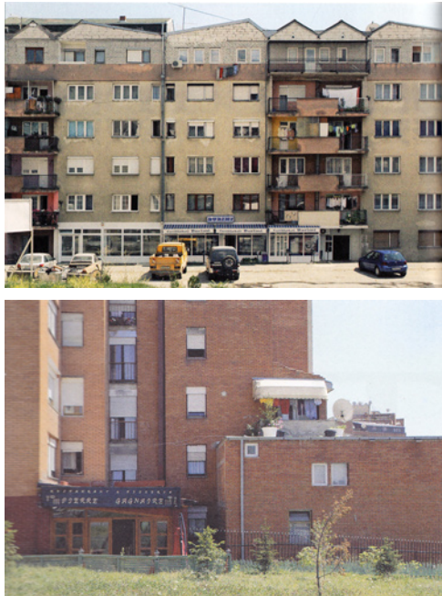
Various kinds of roof appropriations; From: Prishtina is everywhere. Turbo urbanism: the Aftermath of a Crisis (2008)
