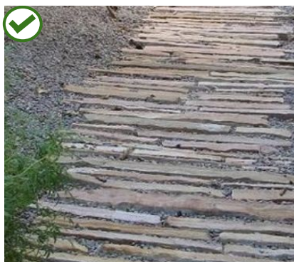
Gravillons / Pierre locale
