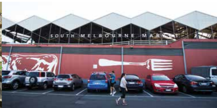
The York Street carpark with our highly visible branding
