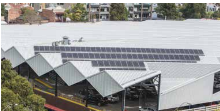
34kW PV solar panels on the Market roof produce 48,580kWh of energy
