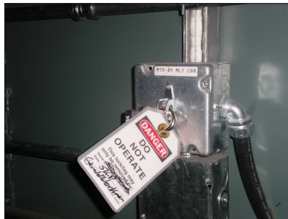
LO/TO AT DOWNSTREAM DISCONNECT (I.E. MOTOR #9)
