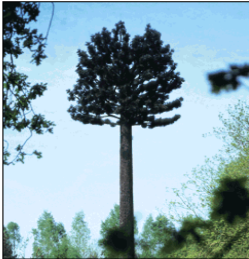
A simulated conifer tree base station, sited harmoniously in an area of natural beauty.
