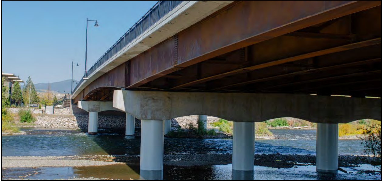
Figure 15: Example Steel Haunched Girder Bridge
