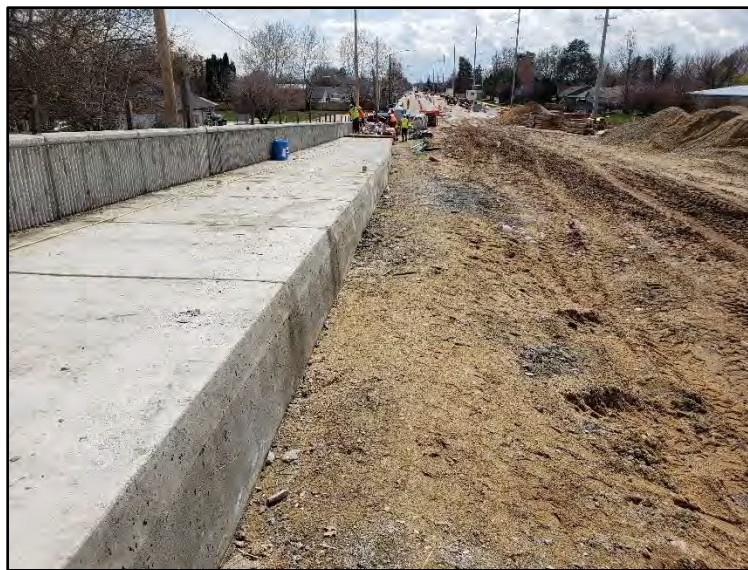
Figure 6: Moment Slab Under Construction
