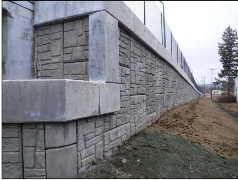
Figure 5: Example MSE Retaining Wall
