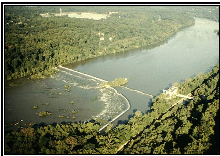
The two dams at Little Falls. The curved dam is Dam #1, a feeder dam for the C & O Canal, the first dam built across the Potomac River. The straight dam is the Brookmont Dam, for water supply in Washington, DC, Arlington and parts of Falls Church, Va. The new fishway is located near the Virginia shore (left to viewer) on the Brookmont dam. Dam #1 is a rubble dam that does not block fish migration.
