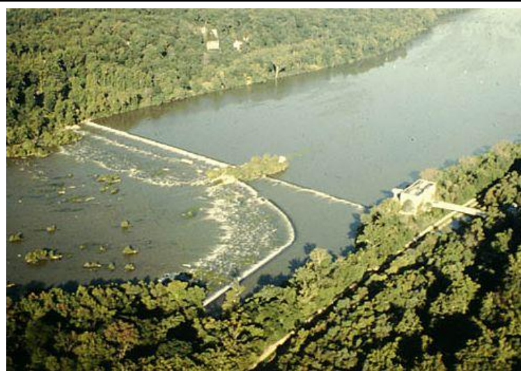
Figure 11: The two dams at Little Falls. The curved dam is Dam #1, a feeder dam for the C&O Canal, the first dam built across the Potomac River. The straight dam is the 1960s Brookmont Dam, used for water supply in Washington, D.C., Arlington and parts of Falls Church, Va. The 2000 fishway is located near the Virginia shore (left to viewer) on the Brookmont Dam. Dam #1 is a rubble dam with enough porosity that it did not completely restrict fish migration. (Image by Curtis Dalpra, ICPRB)
