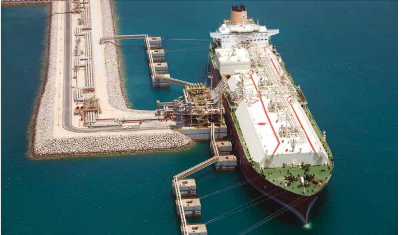
Gas carrier - Ras Laffan Industrial City (RLIC) - Qatar - © GONZALEZ THIERRY - TOTAL
