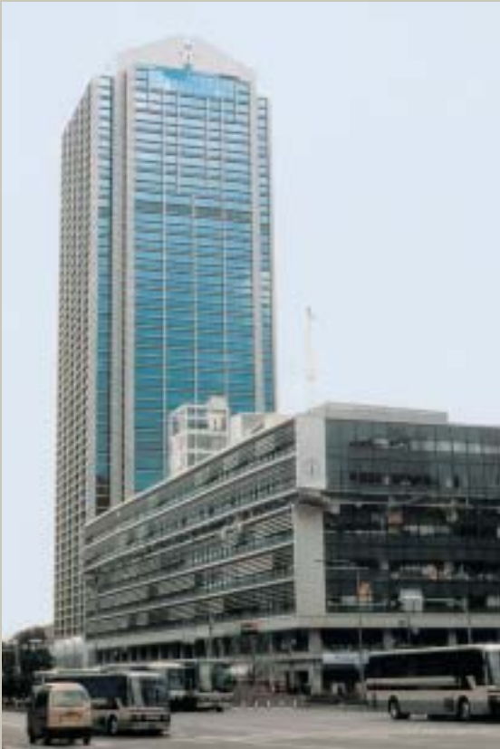
Kobe, Japan, 17 January 2005. The damage to the town hall was typical. The middle storey of the old town hall collapsed. The new high-rise building, erected in accordance with the current building regulations, stood firm.
