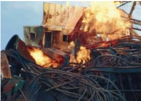
The rig collapses, gas continues to pour out, the heat is enormous. Some five tonnes of steel scrap has to be removed in order to gain access to the blowout preventer.
