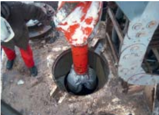
Drilling bit (23-inch) in the bore of the first well.
