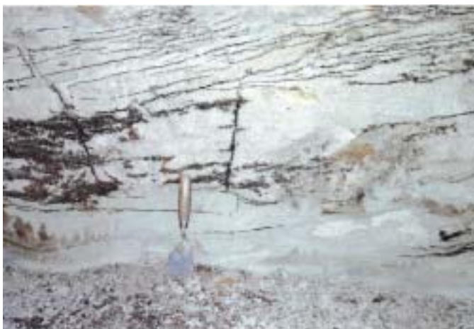
By the time the tar oil (black veins) was discovered to be bound in the sandstone, it was much too late. It was only when the ground was excavated that the tar oil began to flow.
