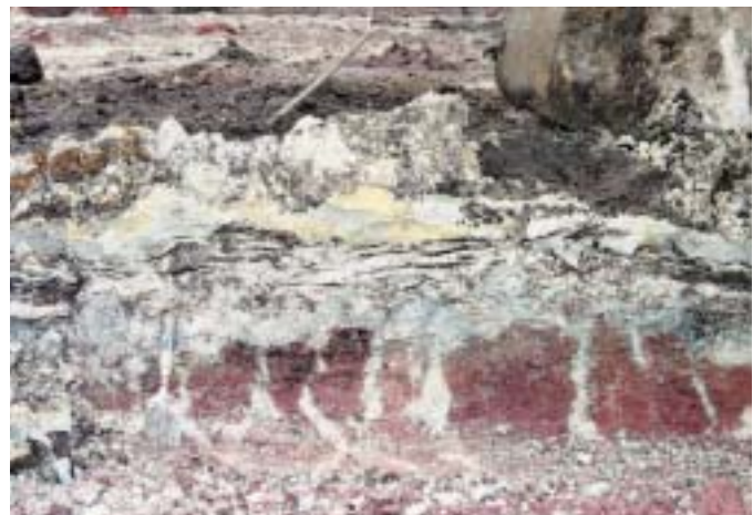
The profile section shows the tar oil contamination in the white sandstone. No-one had expected that the surface of the red mudstone (to the right of the trowel) would also be polluted.
