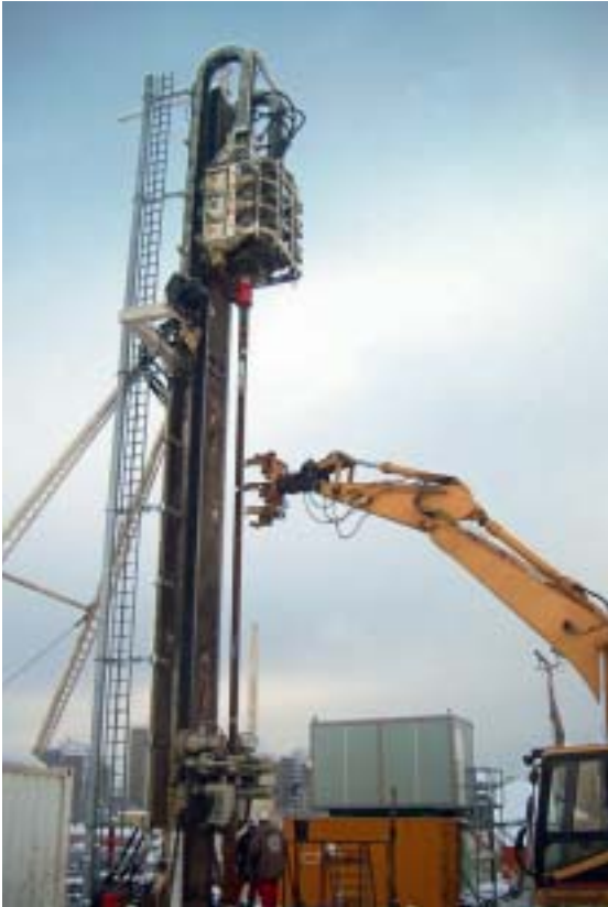
Drilling rig for the first well in Unterhaching.
