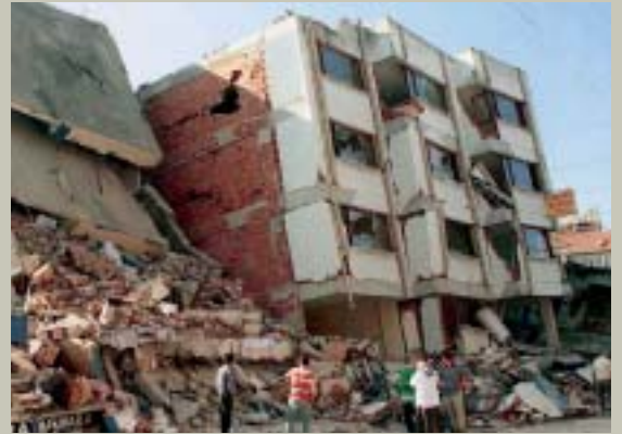
Izmit, Turkey, 17 August 1999. Multi-storey blocks of flats which had been built without adherence to the building regulations suffered the worst damage.
