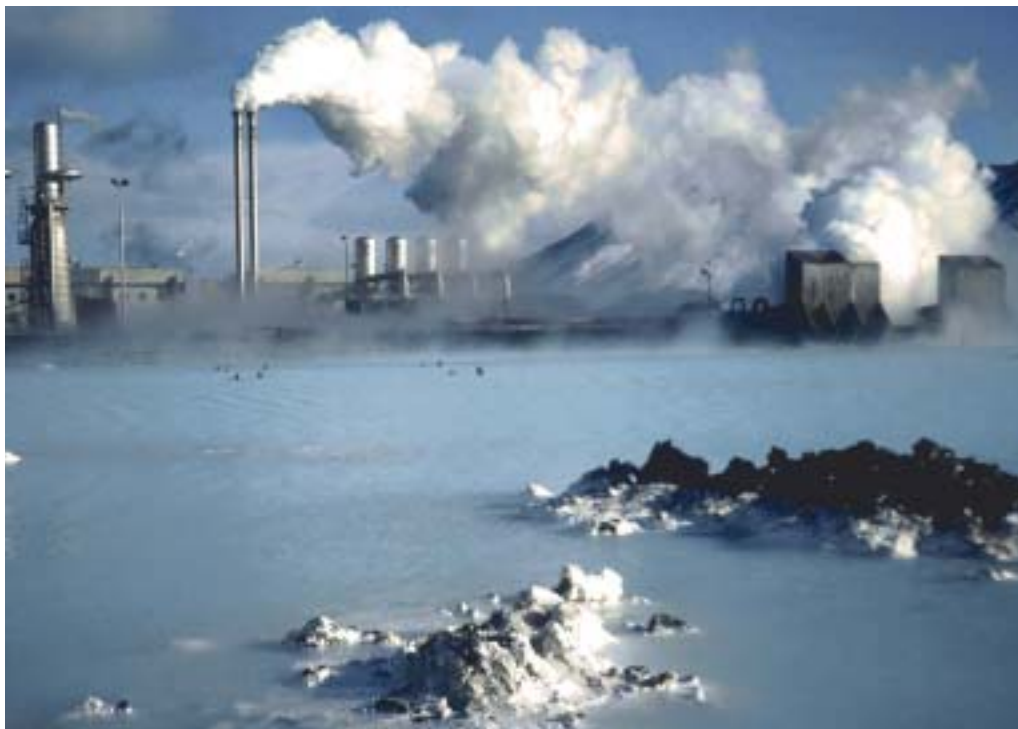
Blue Lagoon, a geothermal power plant in Svartsengi, Iceland. Water at a temperature of about 240°C is drawn from a depth of 2,000 m – a climate-friendly source of energy.
