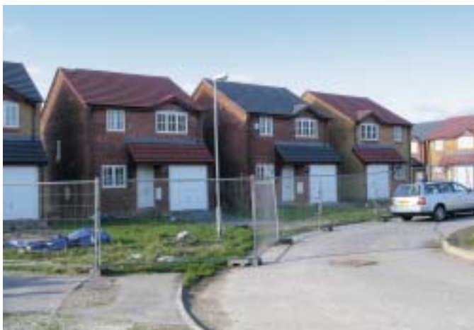
A fence protects the empty houses on the new housing estate. Massive damage occurred because the development plan for the peaty soil did not go far enough.
