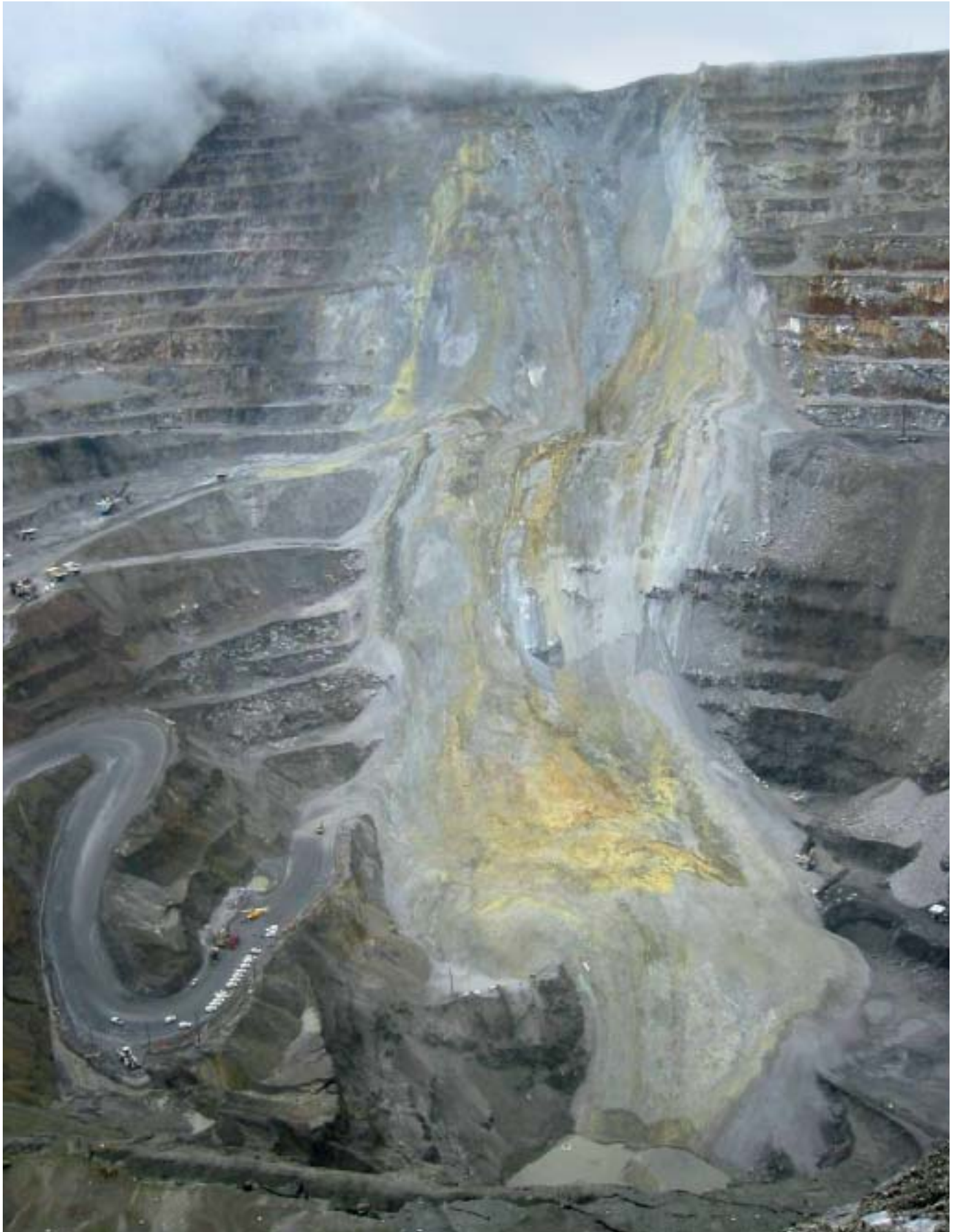
Ore stone slid over 450 m – the length of four-and-a-half football pitches – down to the floor of the mine. The destructive force of the material was immense.
