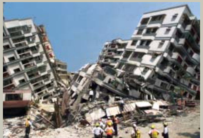
Chi-Chi, Taiwan, 21 September 1999. Numerous apartment blocks collapsed. But the losses caused by incessant power outages were much costlier than those due to structural damage.
