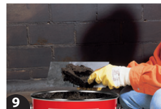
9 After drying the undercoat (about 24 hours) start with the application of the thick coating. To this end, the material is placed on the trowel.
