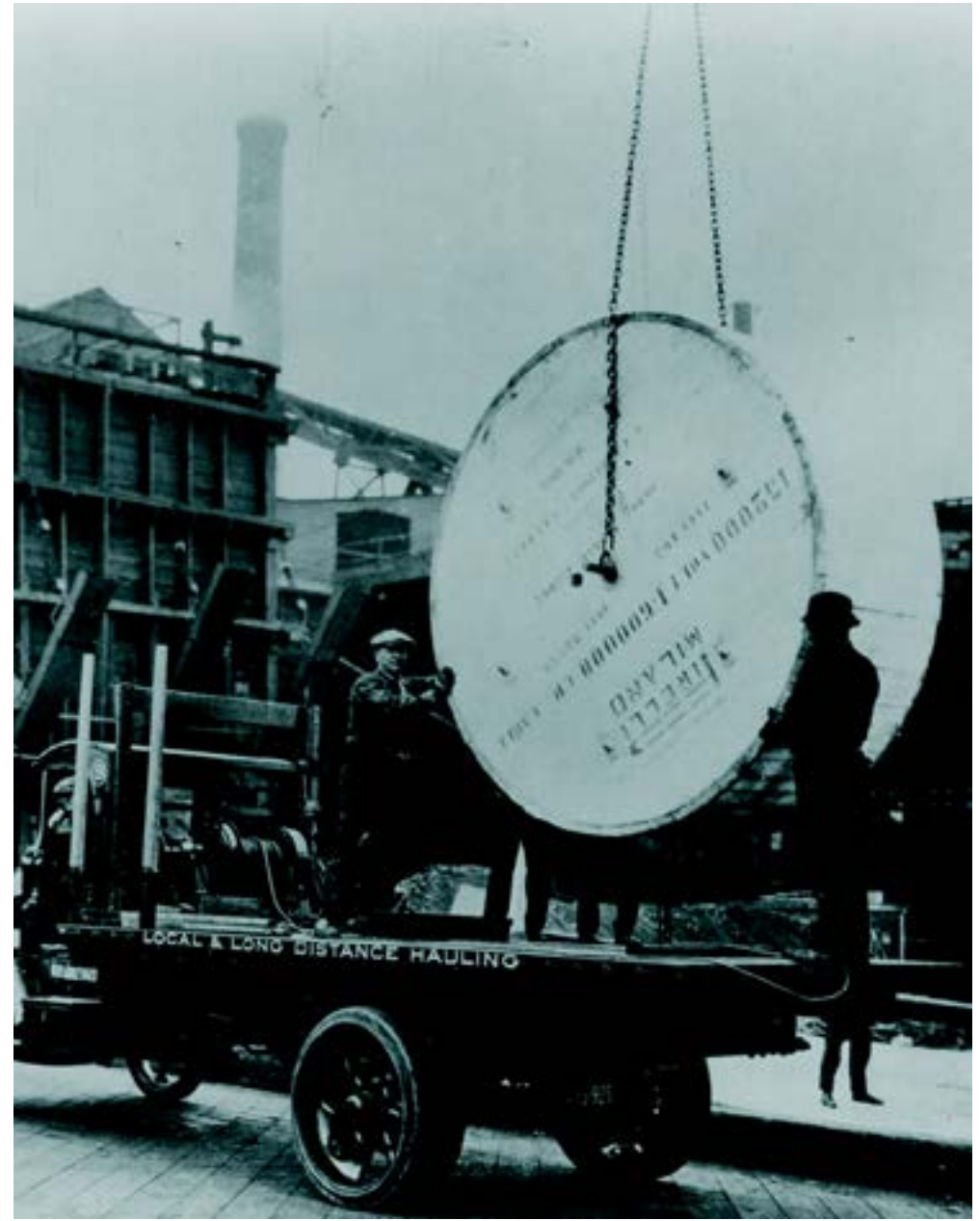
New York, 1927. Oil-filled underground cables manufactured in Milan for the New York metropolitan area's electrical power network being loaded from a barge onto trucks.
