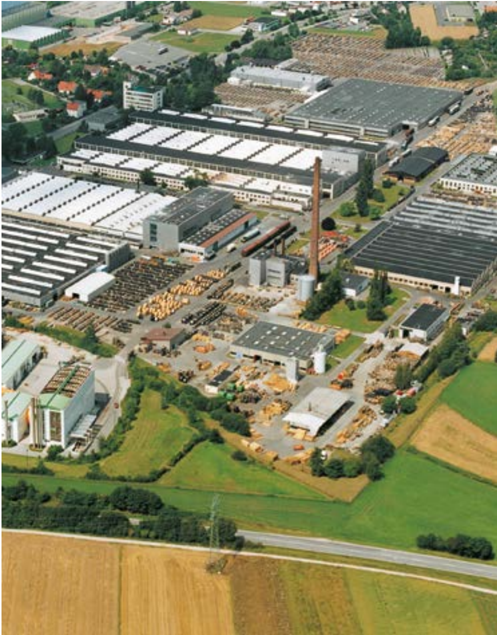
Neustadt plant in Germany producing special cables for industrial applications.
