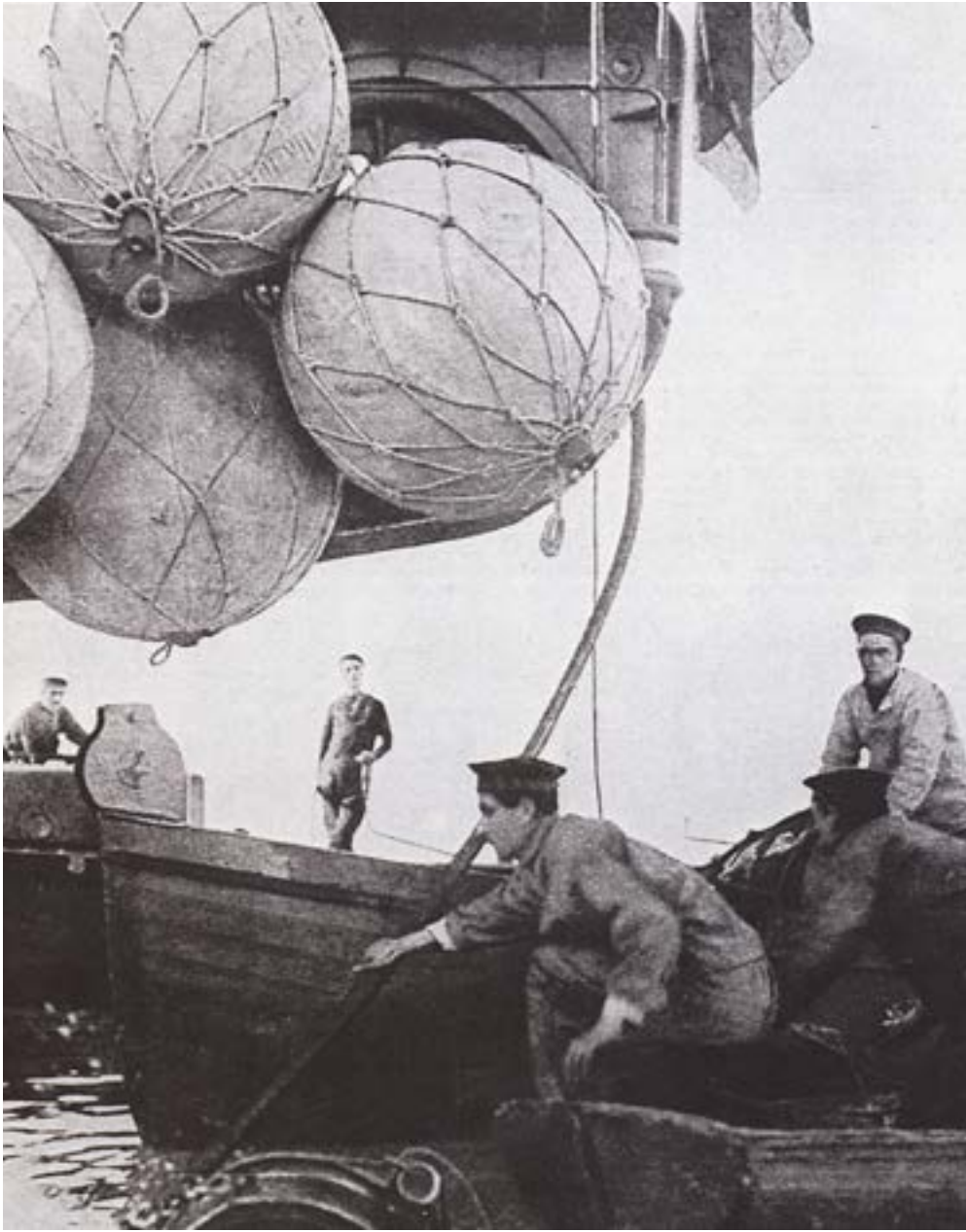
1925, first direct telegraph cable from Italy to America. Laying the cable from the Città di Milano to the town of Anzio.
