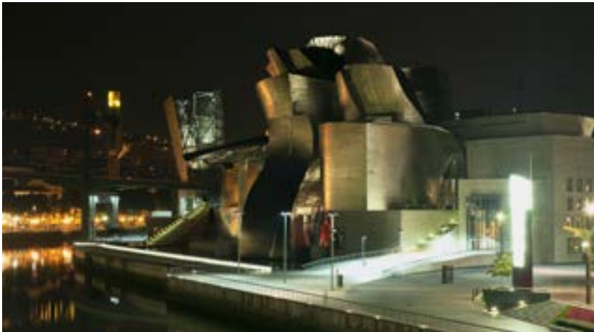
The Guggenheim Museum in Bilbao, equipped with fire-resistant and Afumex cables to reduce smoke and toxic gases in the event of fire.
