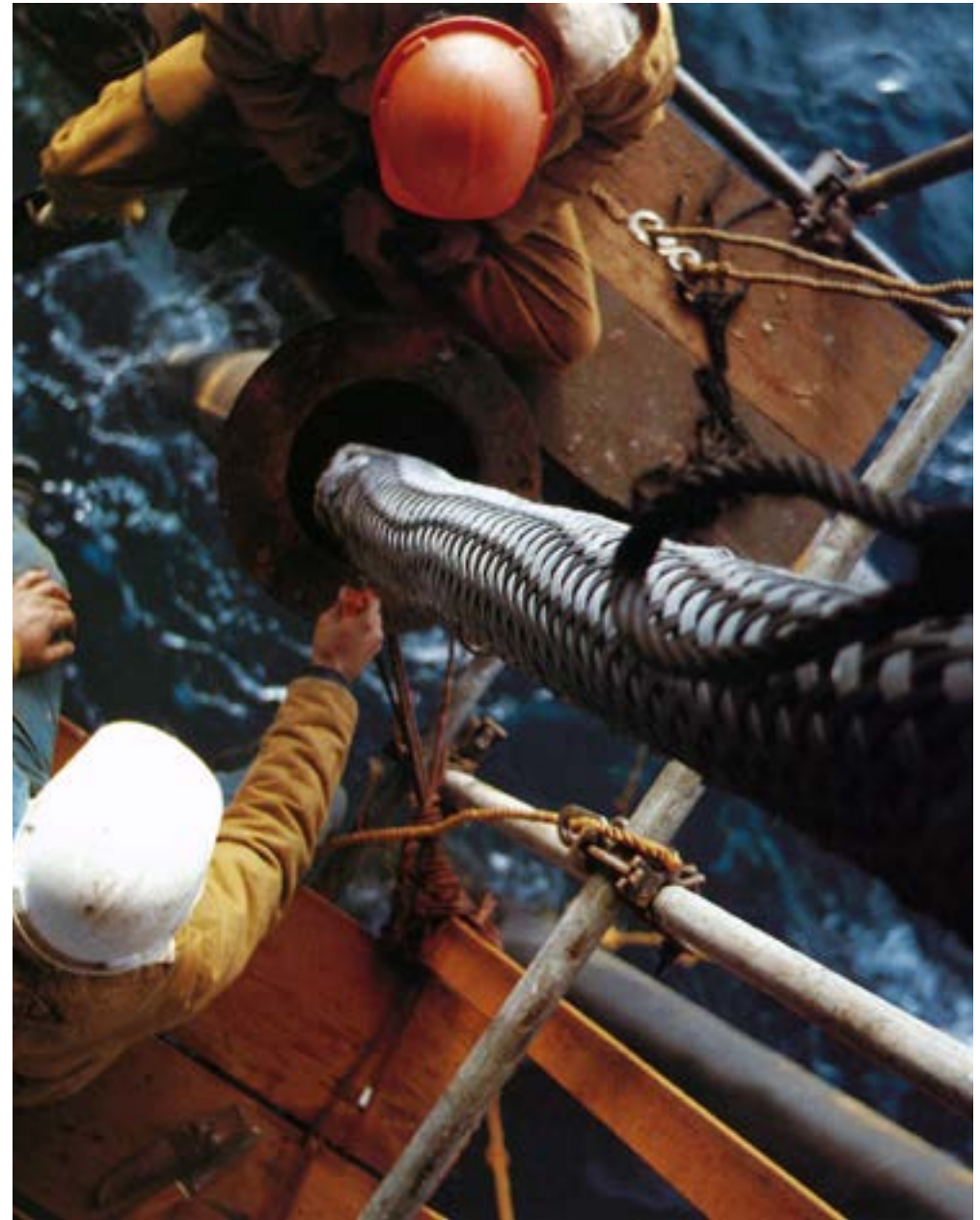
Submarine cable pulling and termination to an offshore platform.
