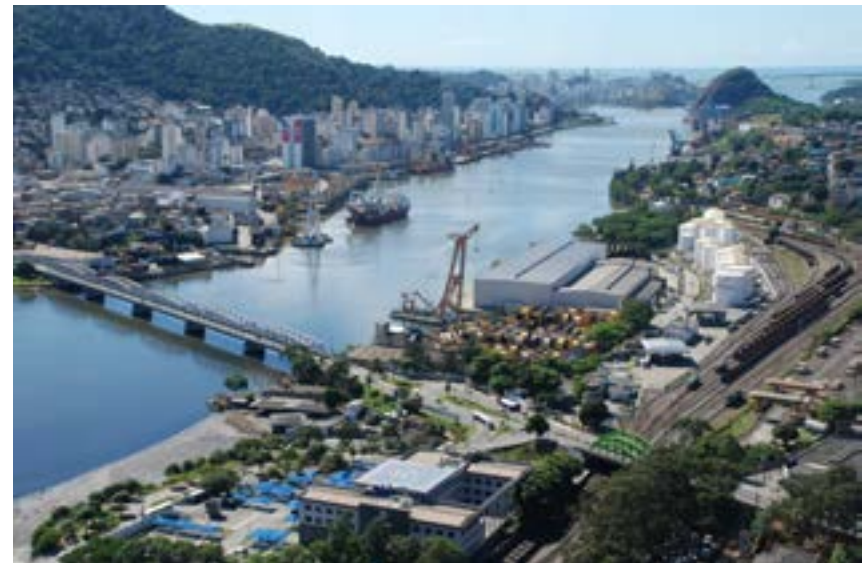
The Vila Velha plant for the production of umbilicals and flexible pipes. Right page: sheathing of the P-Laser® Medium Voltage cable.
