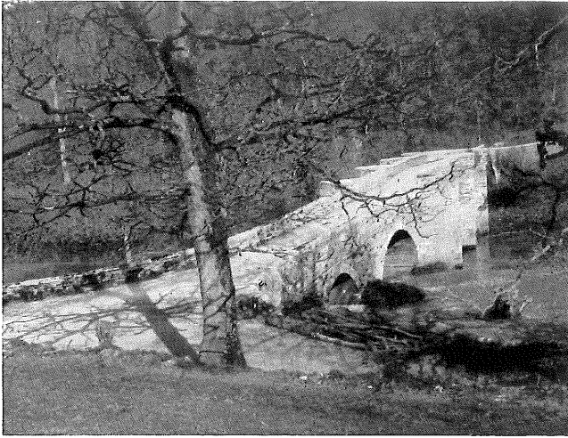
[Photo, H. Coates. Greyston Bridge, over the Tamar. Built 1439.
