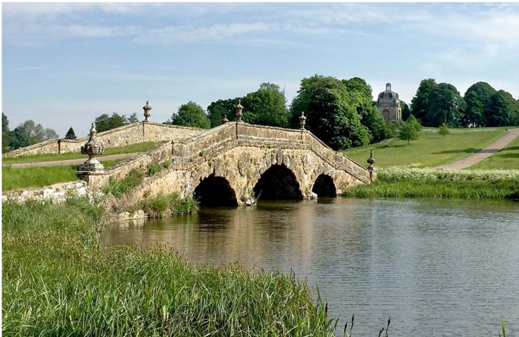
Entrance to Stowe via Bridge Across the Oxford Water with a Boycott Pavilion in View
