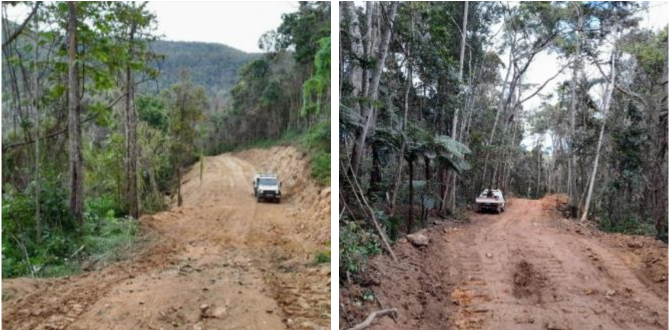
Figure 17: A 5.9km fireline created along a dominant north–south ridgeline in Bulburin NP.
