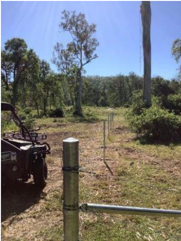
Figure 18: The cattle-exclusion fence (lower images) erected between the park and a neighbouring freehold property to prevent cattle intrusion into Bulburin NP (above).
