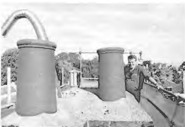
Working on a chimney on the Essex Building.
