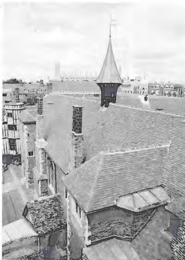
The new roof on Old Hall.
