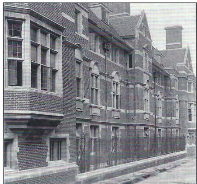
The façade of the Dokett Building on Queens' Lane, c. 1912.
