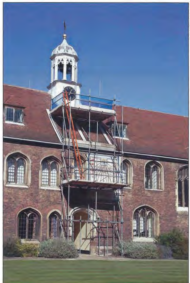
Scaffolding to repair the Clock Tower.
