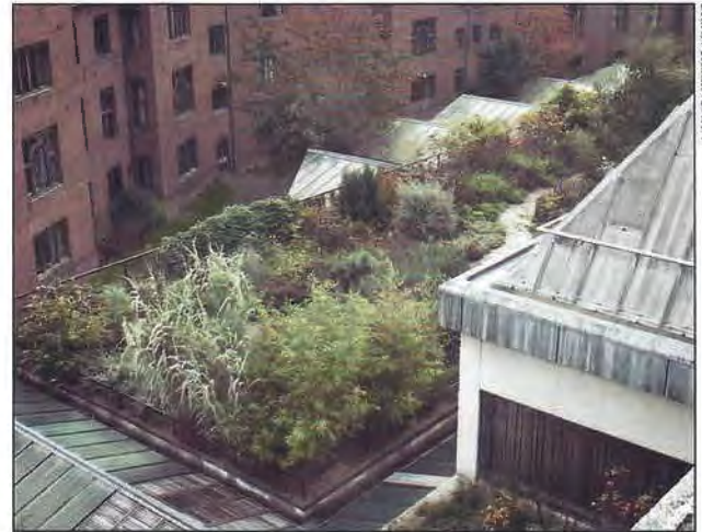
The roof garden in Autumn from the top of AA staircase.
