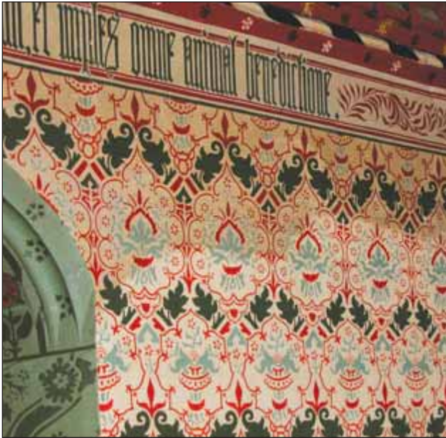
The restoration of the walls in the Old Hall – the line between cleaned and uncleaned is clearly visible.
