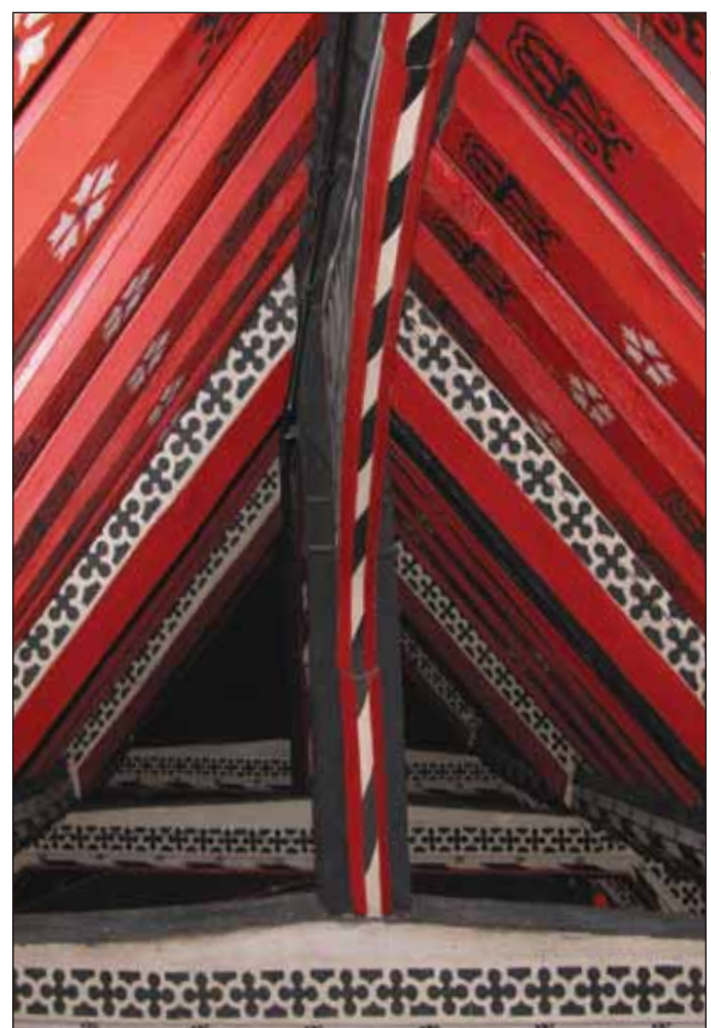
In the eaves of Old Hall during the restoration.
