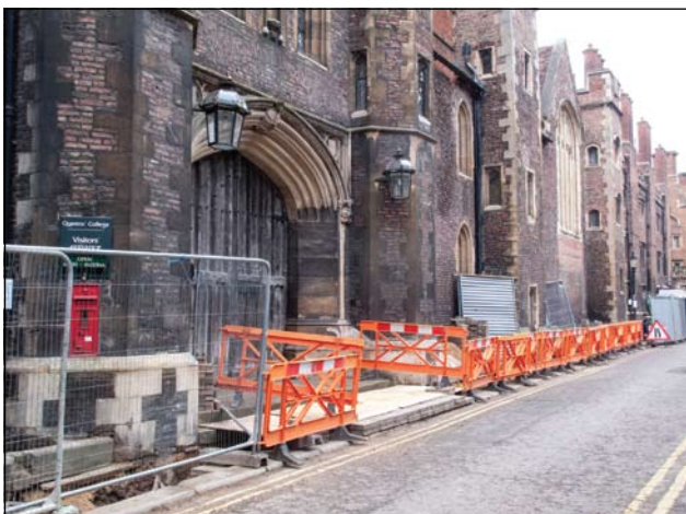
Digging up Queens' Lane for the new electricity cable.
