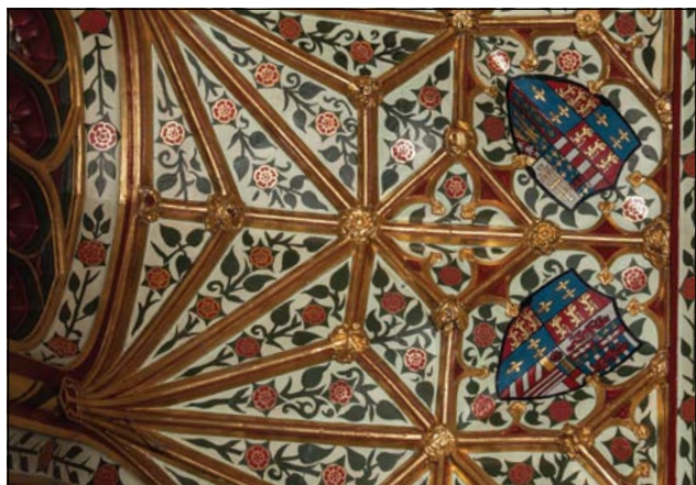
The Oriel Window ceiling, Old Hall.
