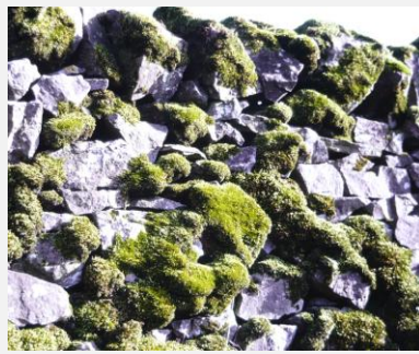
Moss Covered Wall, Winterburn Friars Head, Winterburn, Yorkshire. 34(SD) 936571. March 1989
