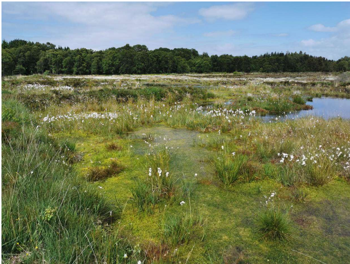
Figure 2.4 Example of existing cell bund constructed at Cloncrow Bog NHA (the vegetation in this photo has developed in the 2 years since cell construction)
