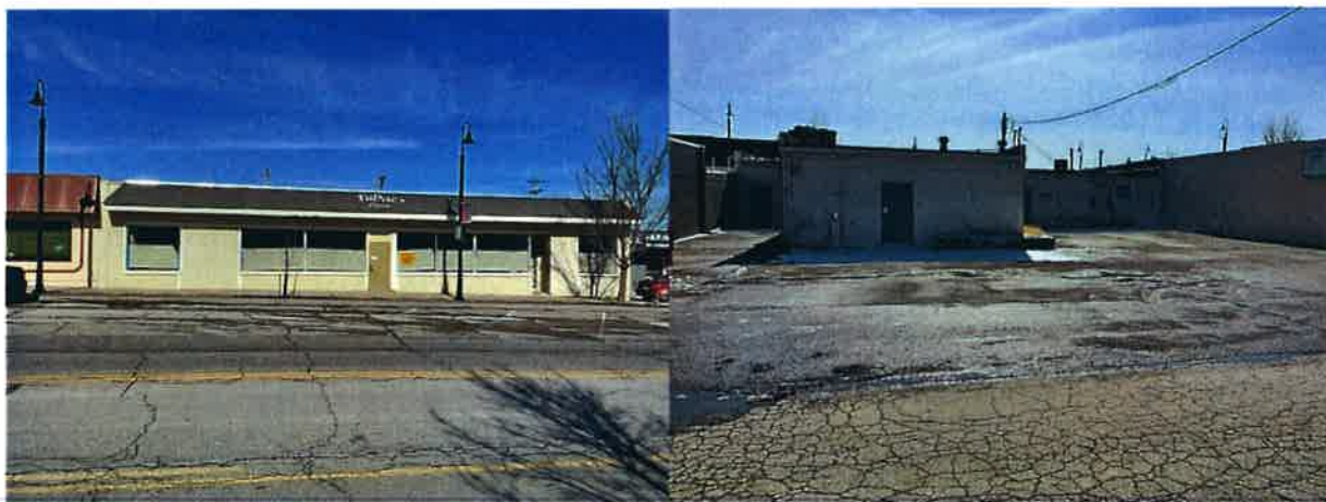
Figure 2 – Site Photos – (L) Storefront on 63 rd Street. (R) Rear of Property on Public Alley
