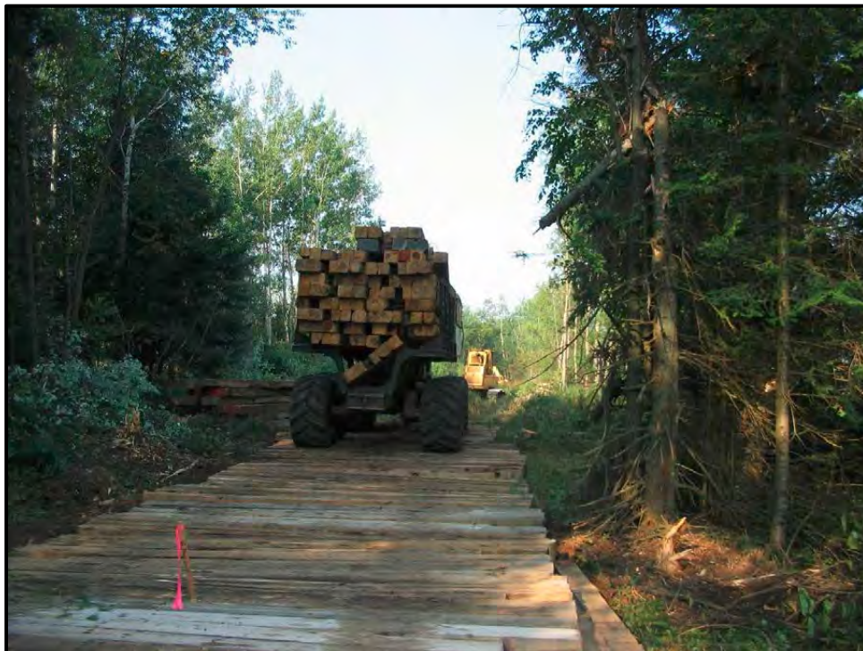
Figure 2.4-8. Timber mats being placed in wooded wetland.
