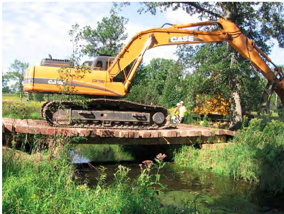
Figure 2.4-9. Timber-mat equipment bridge at a stream crossing.
