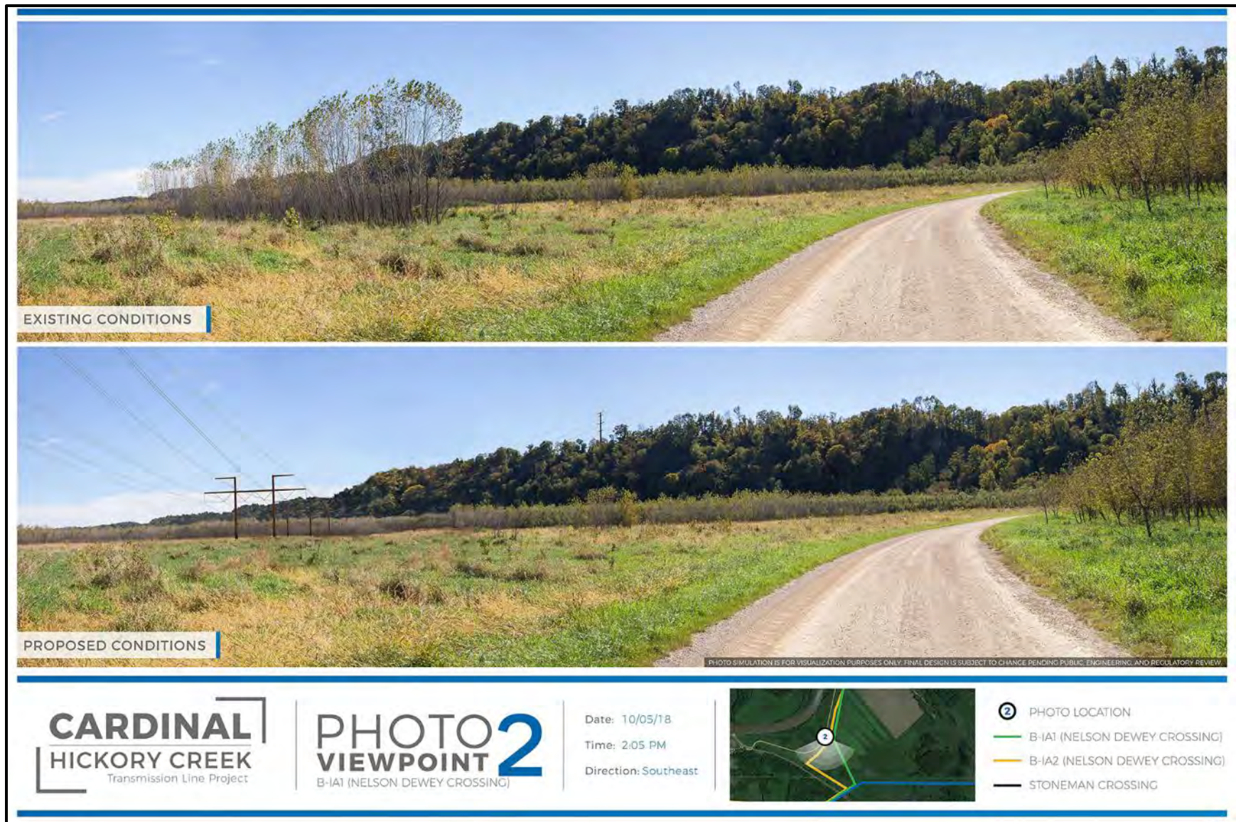
Figure 3.11-16. Visual simulation from viewpoint 2 within the Refuge, on Oak Road (Segment B-IA1).
