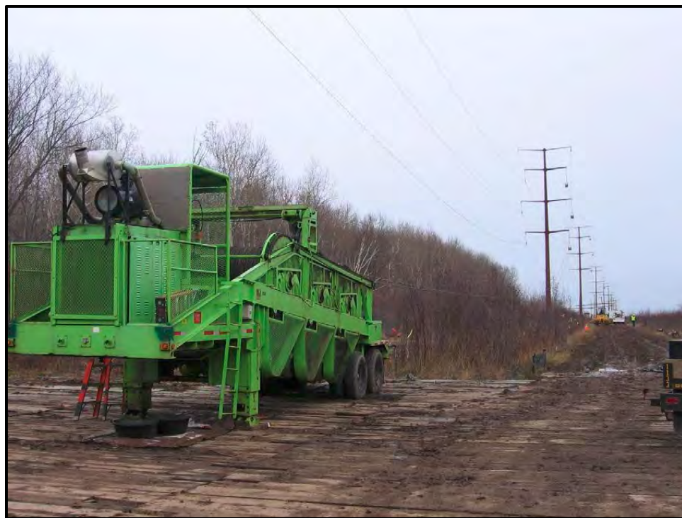
Figure 2.4-14. Pulling the conductor through the structure arms.
