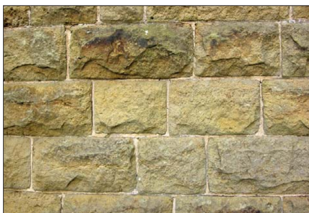
Picture 16. Victorian coursed rockfaced sandstone
