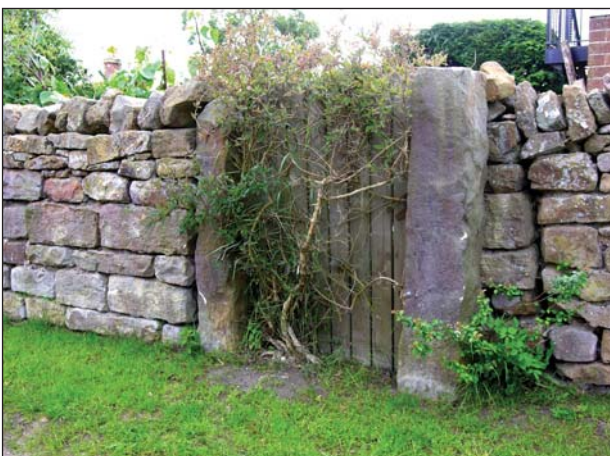
Picture 24. Traditional roughly hewn stone Gate Posts
