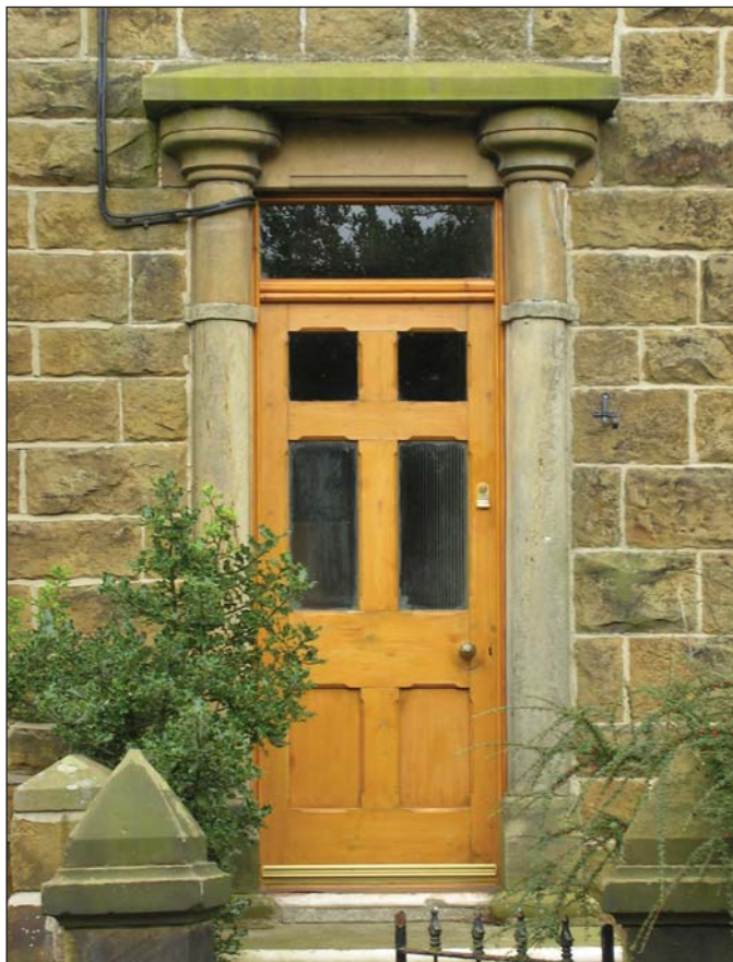
Picture 30. Victorian panelled door in unusual stone doorcase
