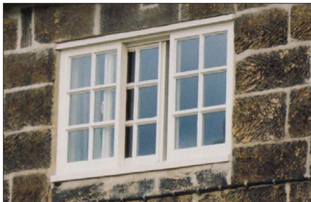
Picture 7. A traditional "Yorkshire" horizontally-sliding sash window - once a typical feature of older buildings in Moorsholm
