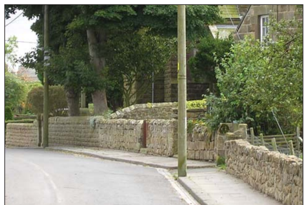
Picture 19. Stone boundary walls - important characteristic features
