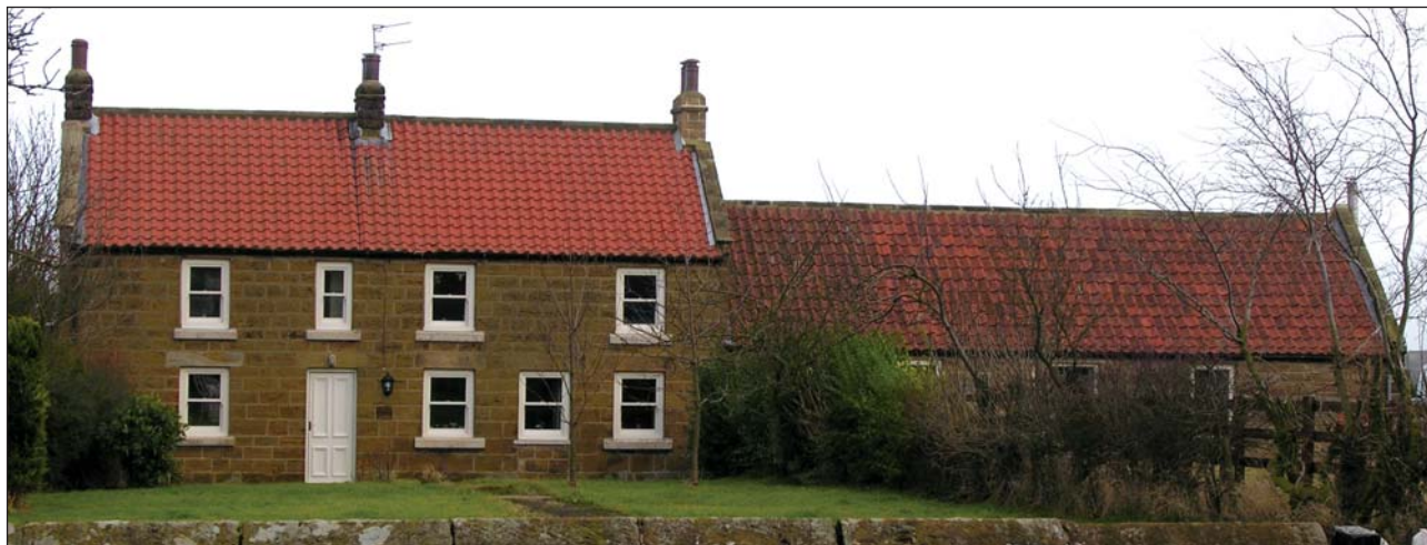
Picture 38. Characteristic stone-built victorianised vernacular farmhouse with pantiled roof and timber windows and door
