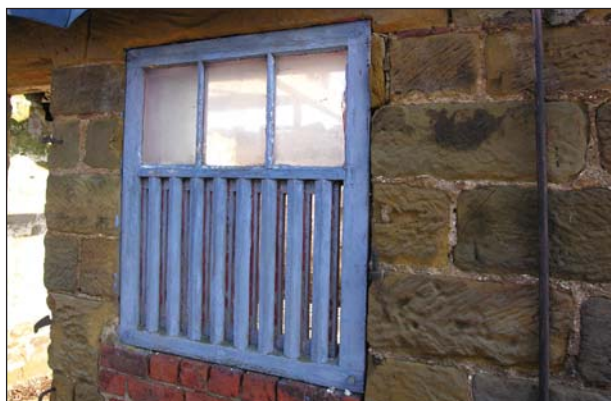
Picture 9. Traditional stable window - part glazed, part "hit-and-miss"
