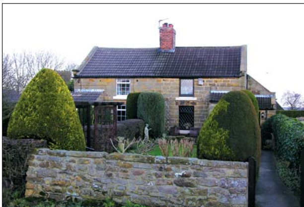
Picture 12. Old Quaker Meeting House on the back lane
