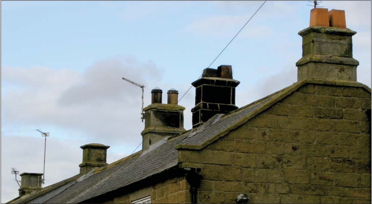
Picture 5. Pitched roofs articulated by chimney stacks with clay pots
