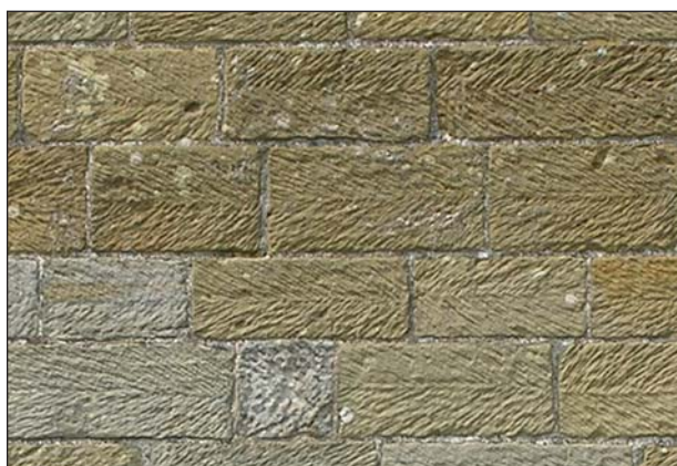
Picture 15. Traditional herringbone dressed sandstone
