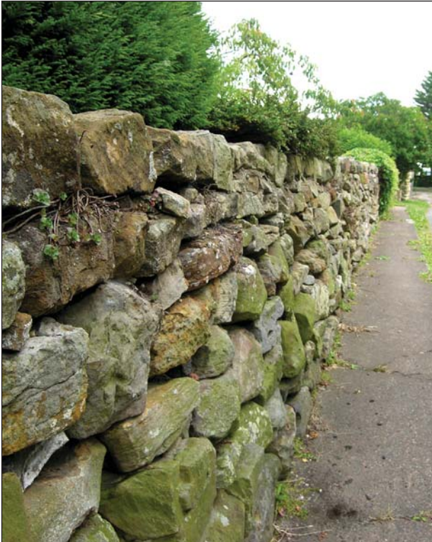
Picture 17. Characteristic drystone wall
