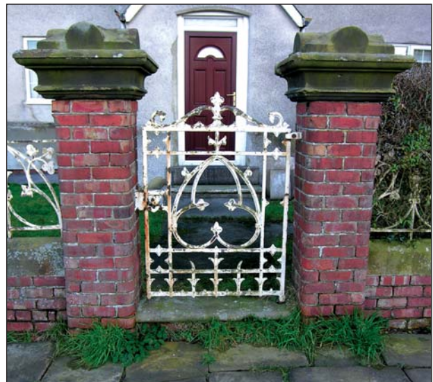
Picture 18. Attractive Victorian iron gate and brick and stone gatepiers
