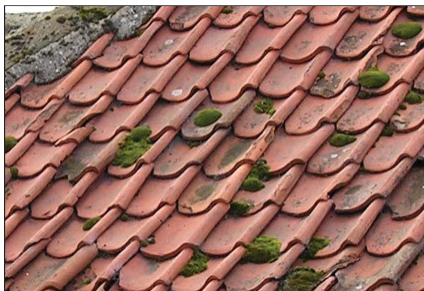
Picture 14. Roof clad in authentic traditional clay pantiles
