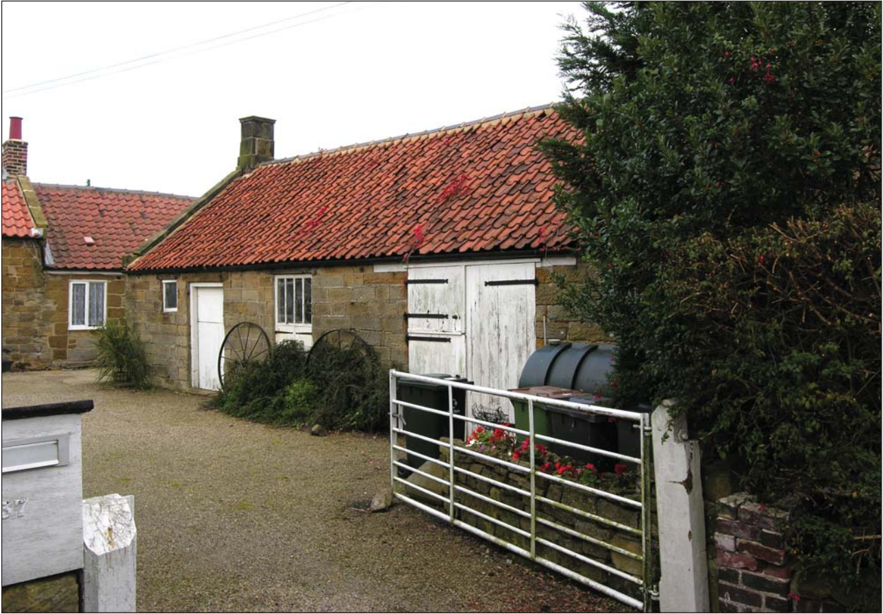
Picture 1. The Forge, Moorsholm's only listed building
