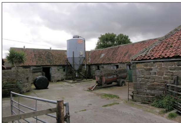
Picture 8. Traditional farm buildings with stonewalls and clay pantile roofs
