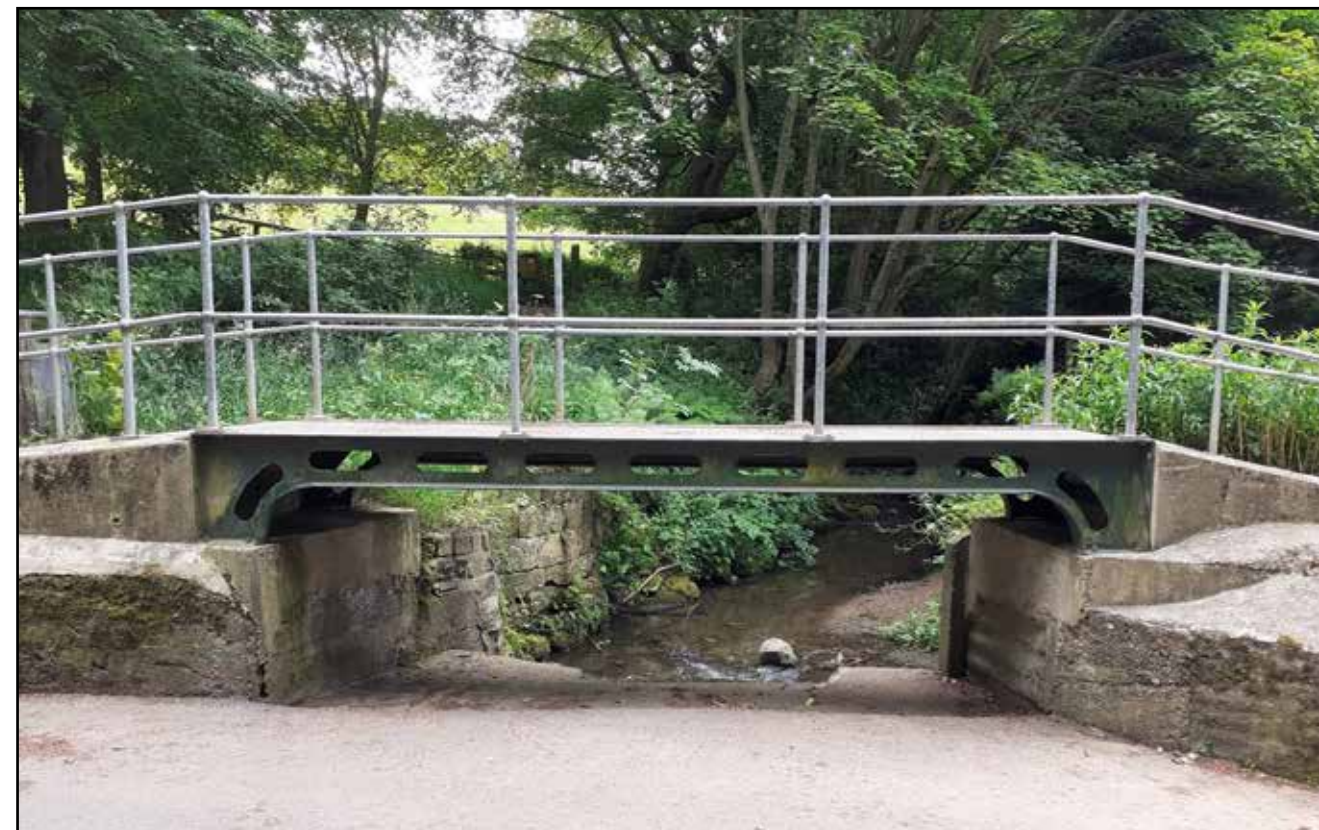
Unsympathetic steel bridge and railings, Dam Street
