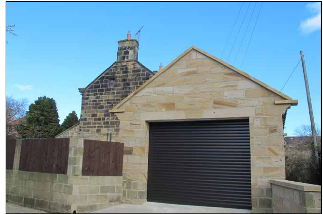
New garage reflecting traditional character and materials
