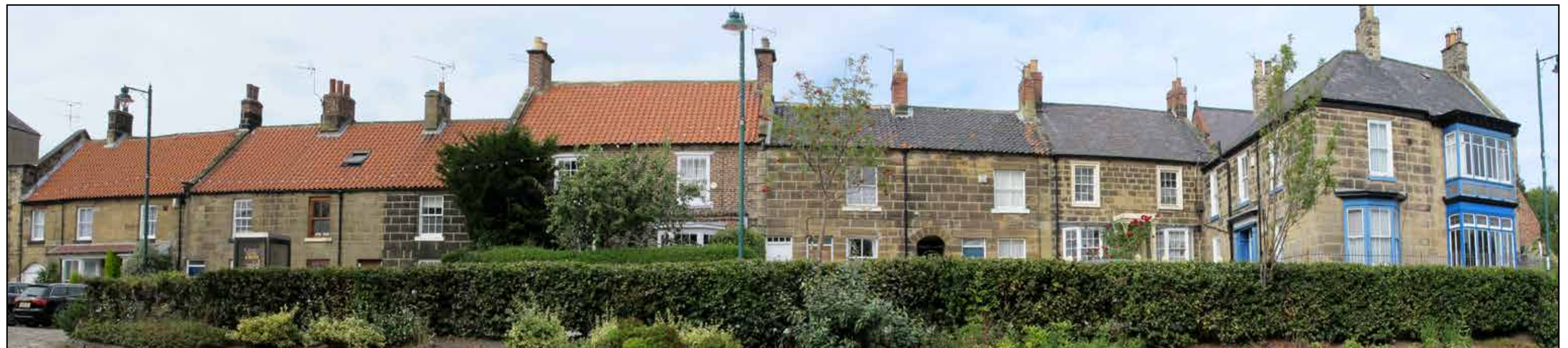
Grey concrete roof tiles contrast with the mature patina of natural clay and slate roofscapes
