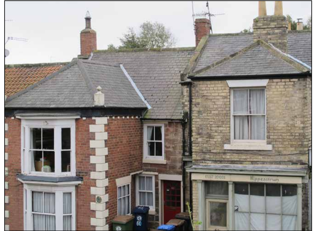
Sliding sash windows in Loftus, both vertical and "Yorkshire" horizontal types. Some are likely to be original pitch pine which if maintained properly can last indefinitely
