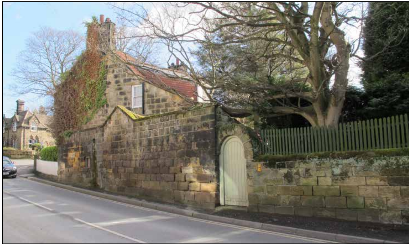
Historic Listed Wall, Jessemine Cottage
