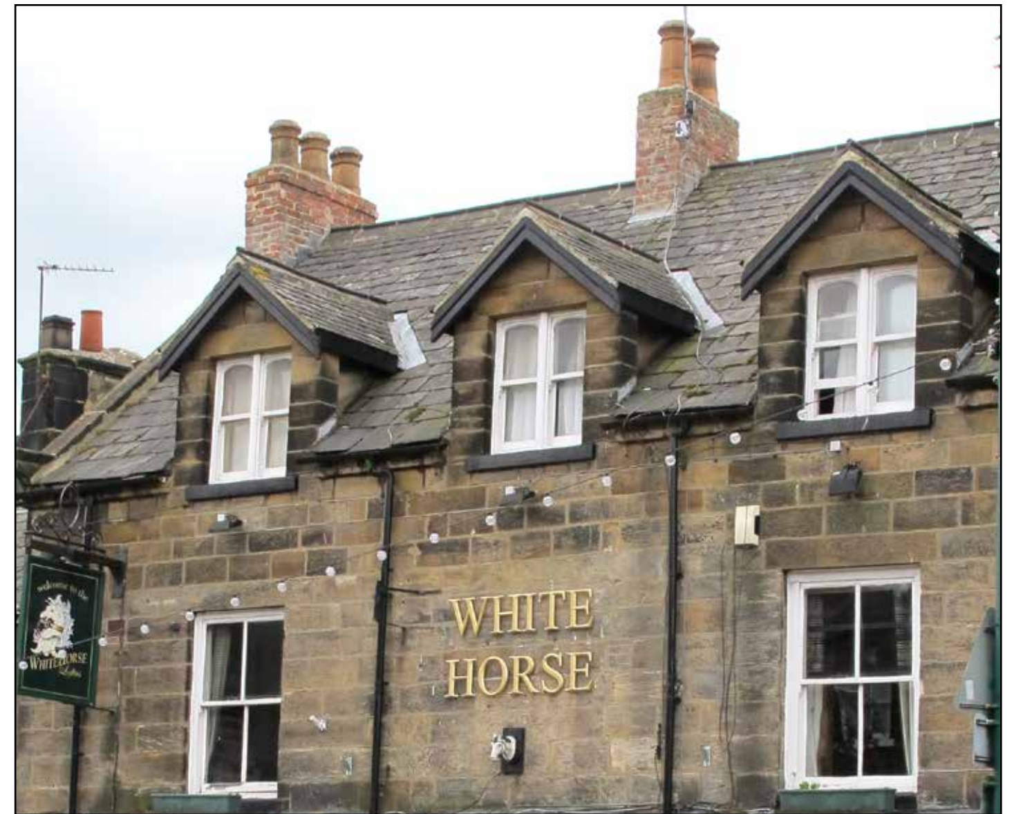
Integral correctly proportioned dormer windows
