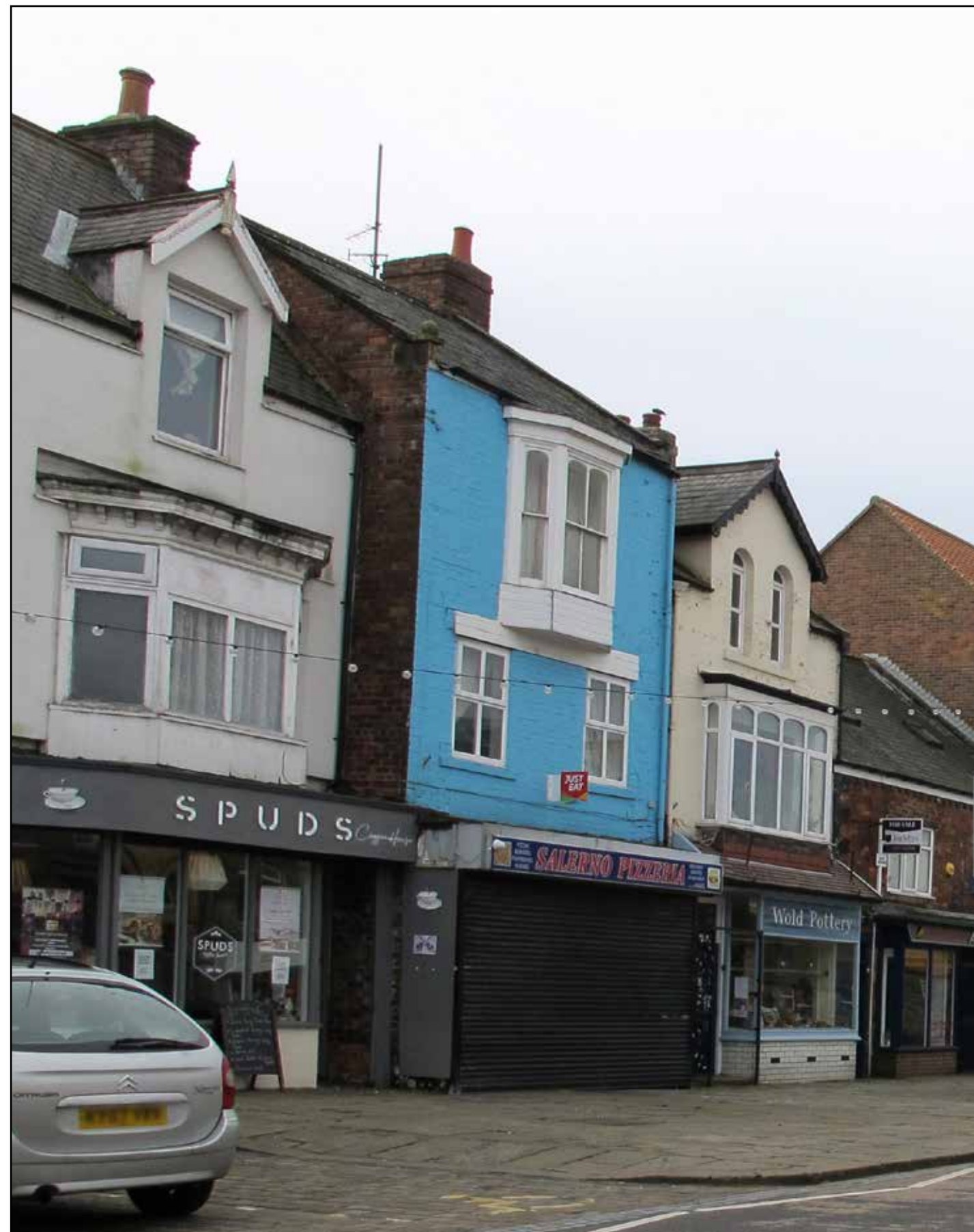
Obscured Facing Materials, Loftus Market Place
