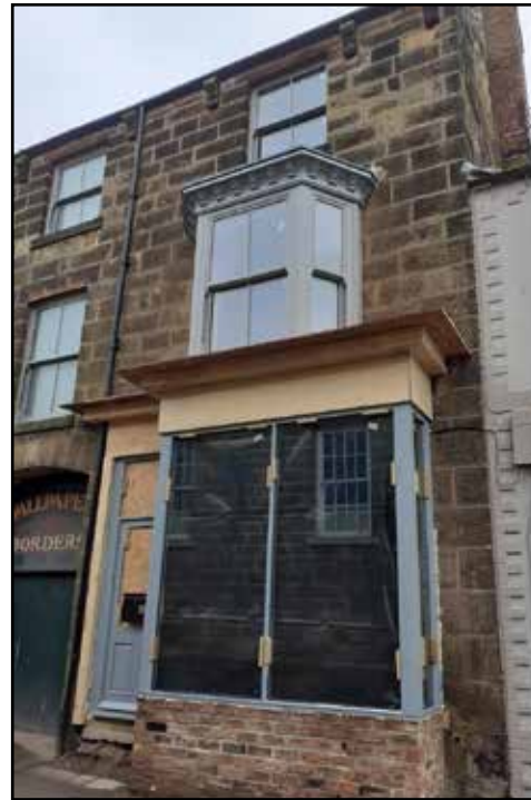
Re-introduction of traditional proportioning and sliding sash windows, North Road.
