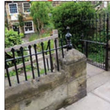
Boundary Wall, Gatepiers, Gate and Railings to south of NO. 19 Grade II - 1312758
