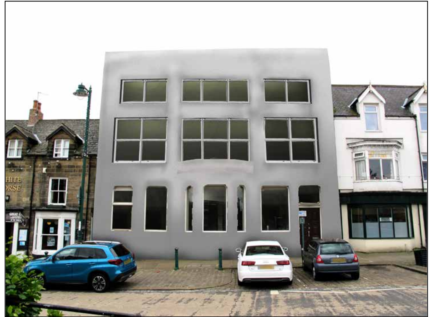
Modified image showing harmful alterations to the façade of a classical building
