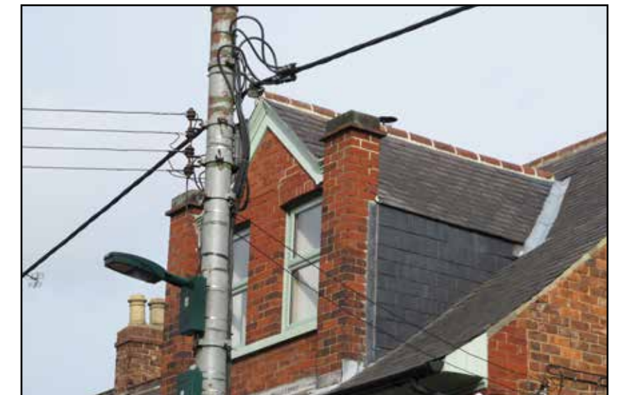
Intrusive infrastructure, Zetland Road
