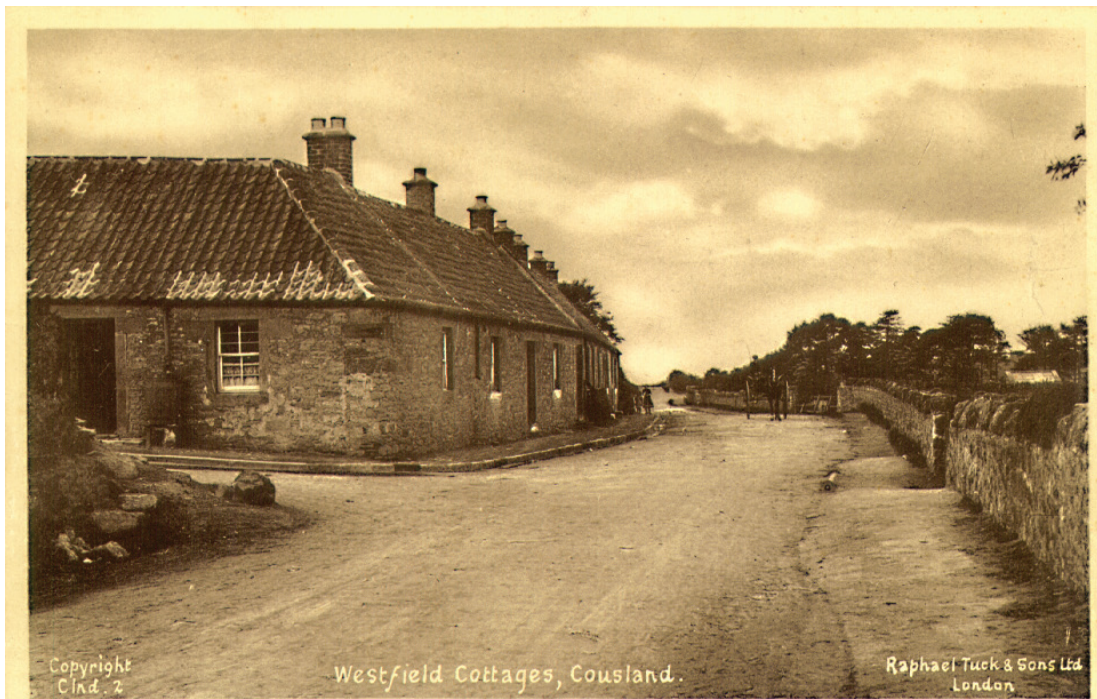
Fig. 5 A postcard showing Westfield cottages, Cousland, 1901. (Reproduced courtesy of the Cousland Local History Project)
